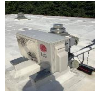
Ductless mini-split HP
