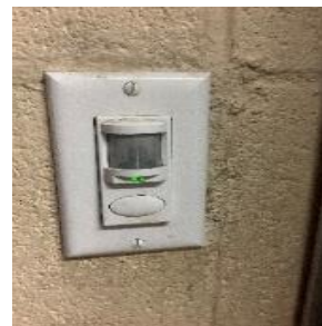
Wall-mounted occupancy sensor
