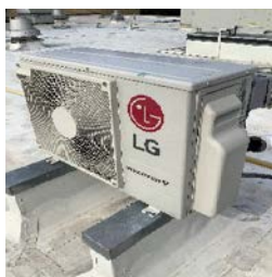
Ductless mini-split HP
