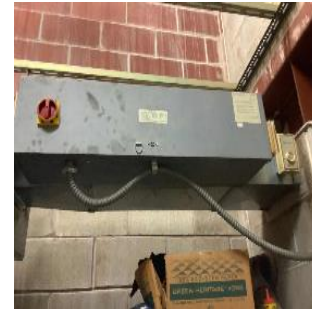
Electric unit heater
