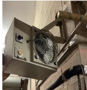
Electric unit heater
