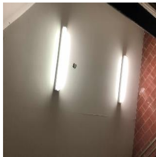
Fixture with 4' T8 tubes
