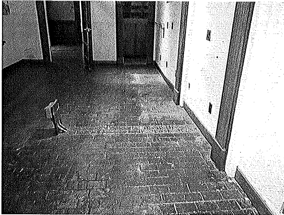
Original first-floor flooring, wood block over creosote
