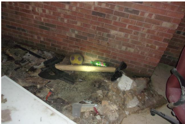
ACM floor debris in hallway areas
