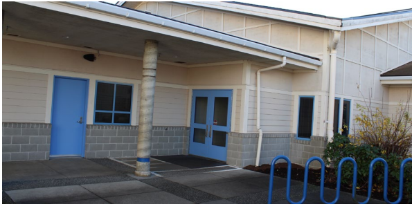
Access control system with lockdown functionality on exterior doors
