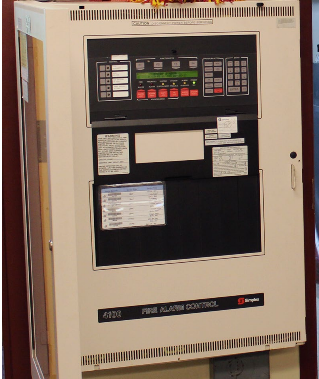
Replace fire alarm control panel
