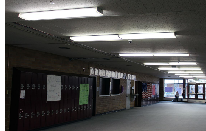
Update light fixtures to energy-efficient LEDs
