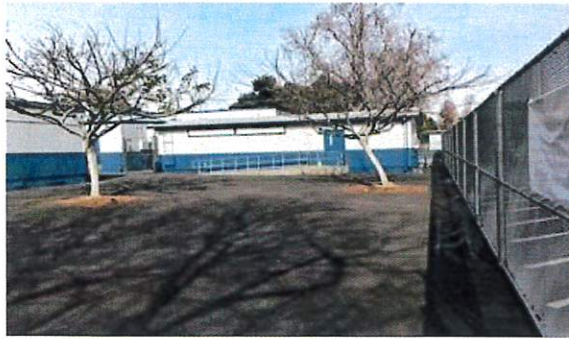
Bret Harte portable #23 Modernization including new siding, paint, flooring, restroom upgrades and 21st Century Technology upgrades
