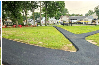
New walkways at Franklin School.
