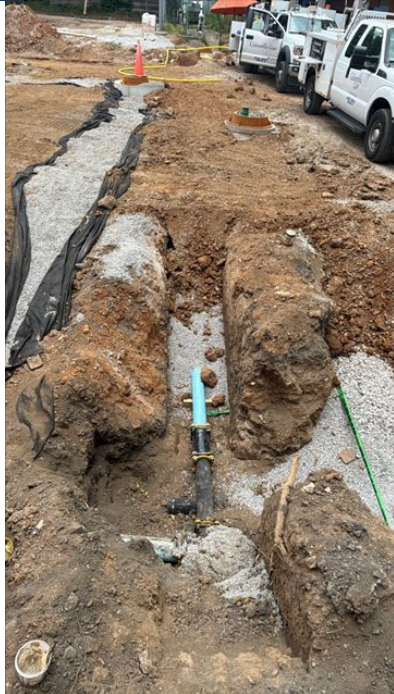
New Fire Main Installation
