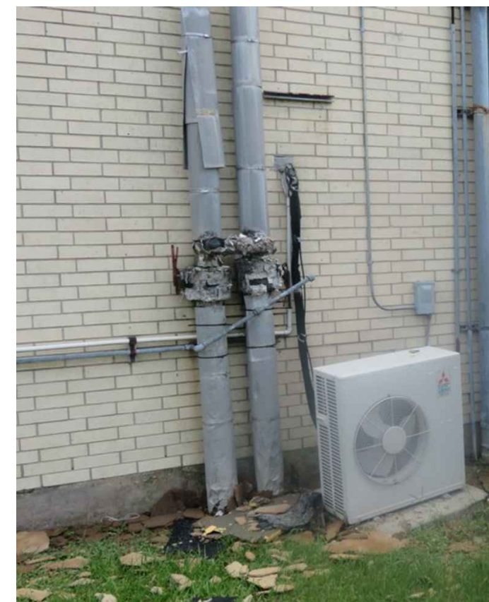
16 Zone 1 - Building G - Picture #1 N.T.S.
