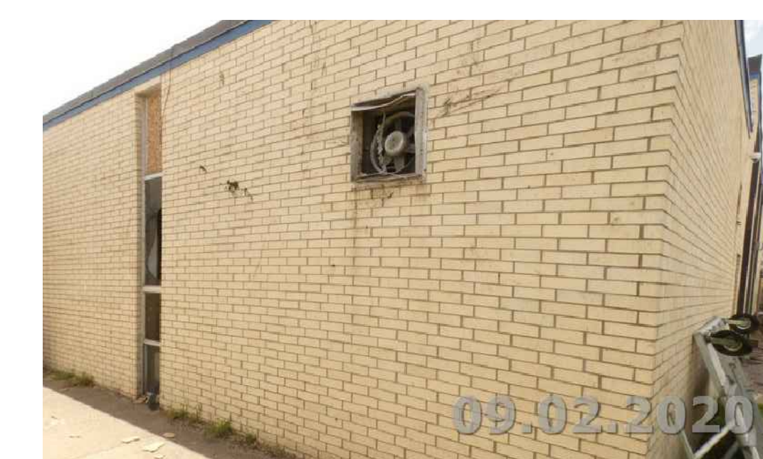
19 Zone 1 - Building G - Picture #4 N.T.S.
