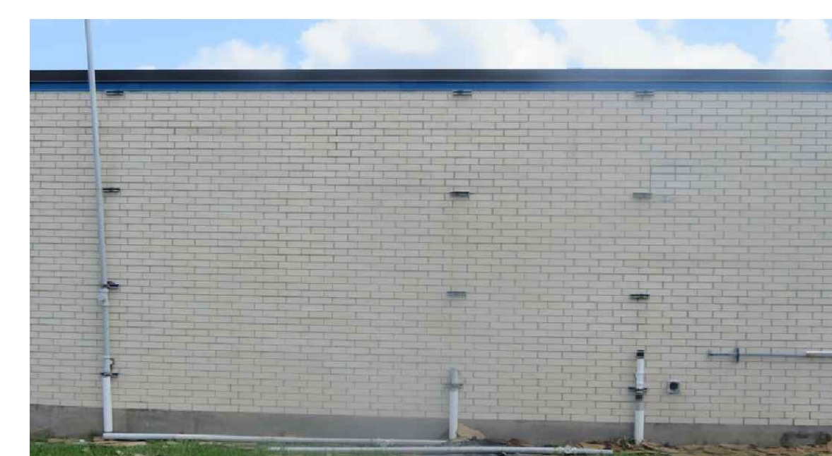
18 Zone 1 - Building G - Picture #3 N.T.S.
