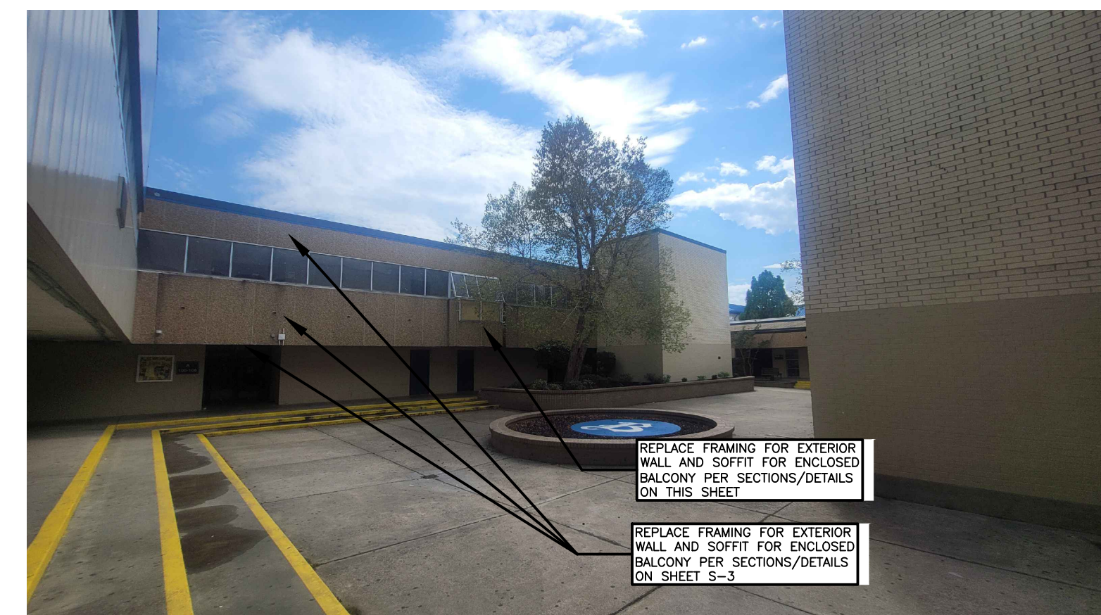
A ENCLOSED BALCONY (w/ ALCOVE) AT BUILDING A SCALE: NOT TO SCALE
