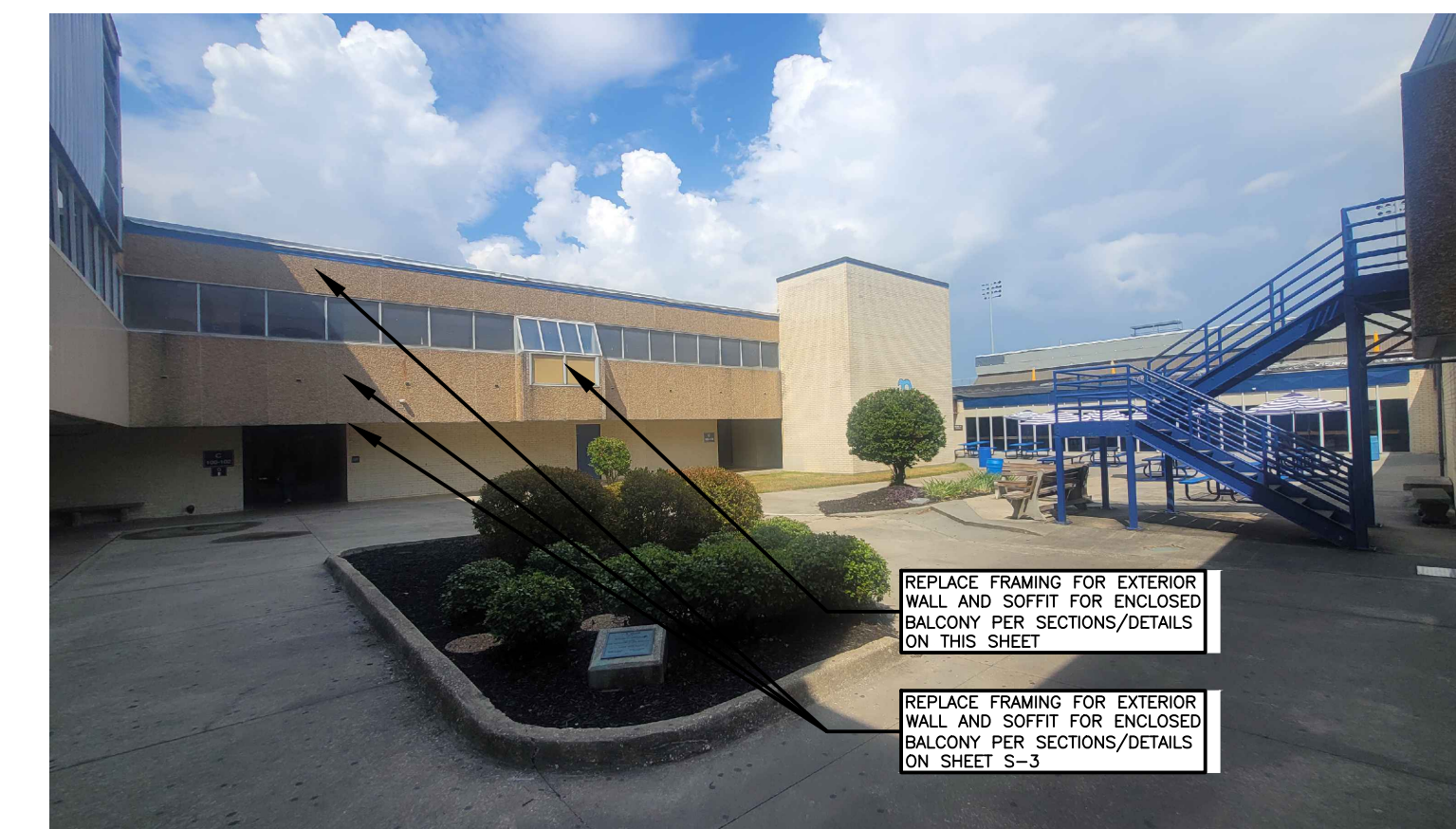
C ENCLOSED BALCONY (w/ ALCOVE) AT BUILDING C SCALE: NOT TO SCALE
