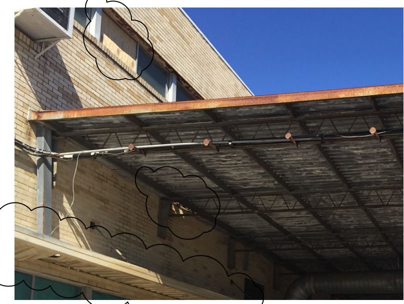
EXTERIOR PHOTO 555: EXISTING ALUM WINDOW & MTL ROOF
