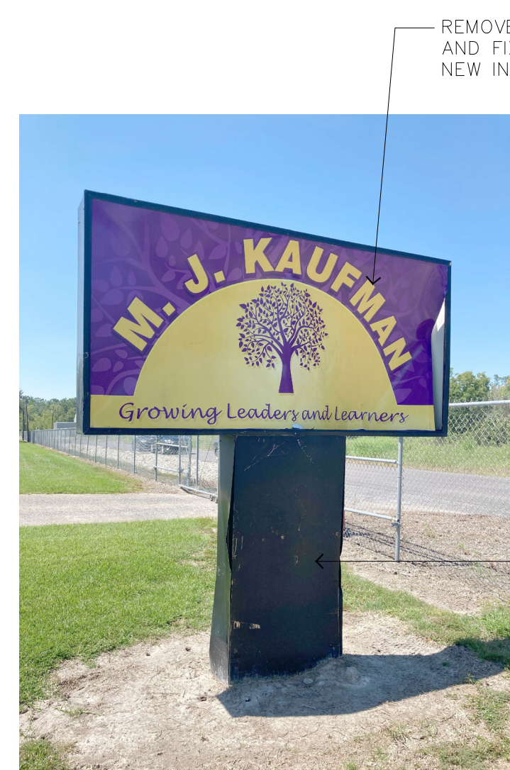
17 Existing Photo No Scale Exterior Photo
