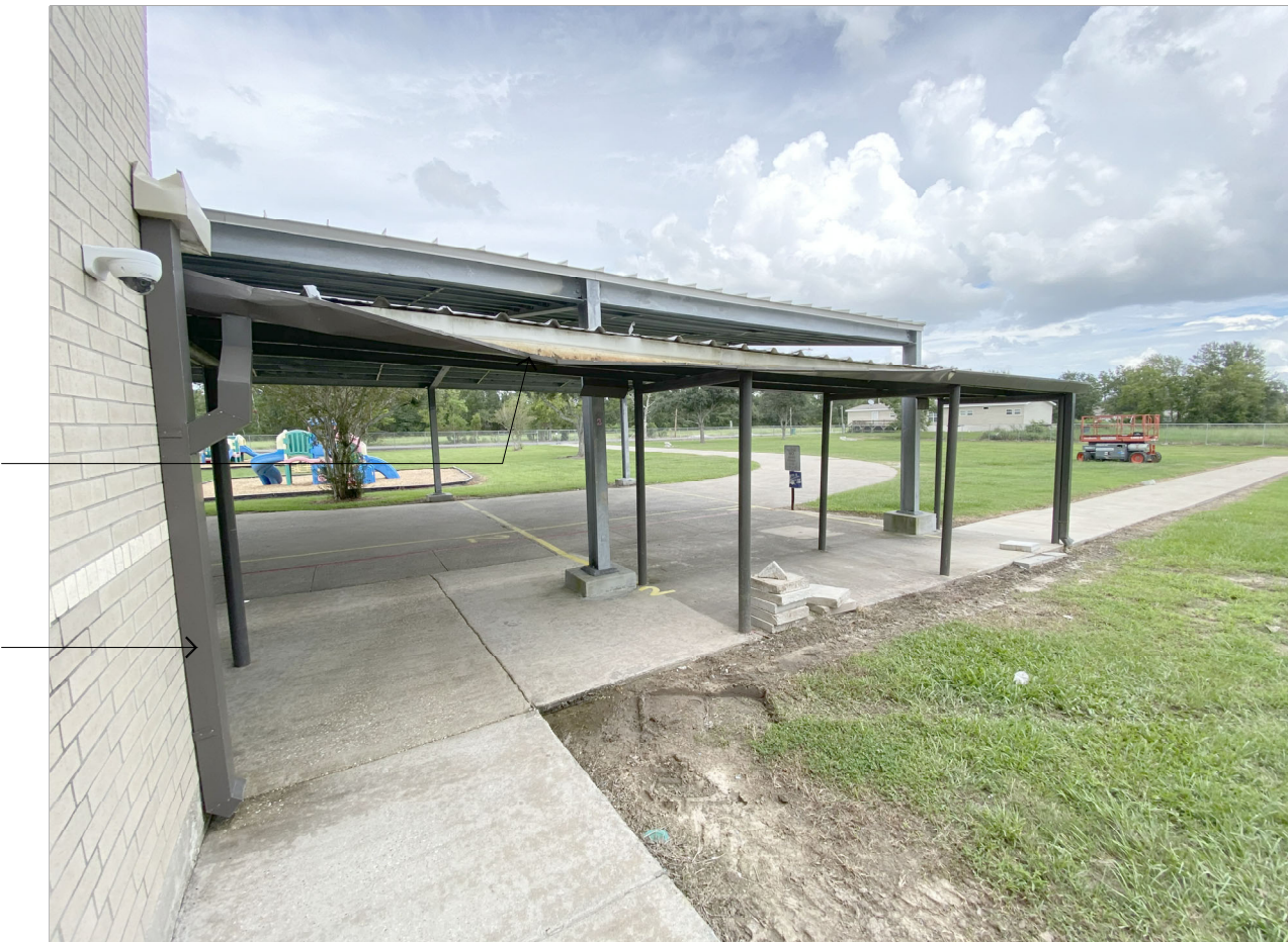
15 Existing Photo No Scale Exterior Photo
