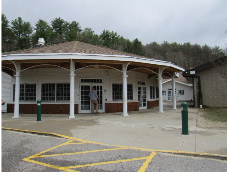
View of Community Center entrance
