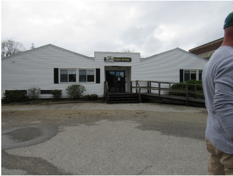
View of non-public entrance between portable classrooms.
