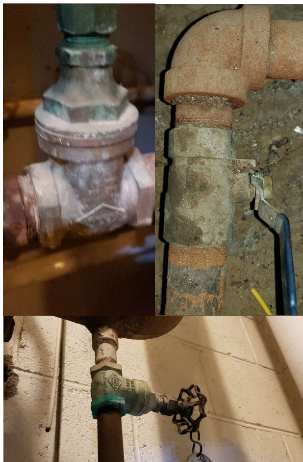
Pipe Elbows, Tees, and Connector – Lead Containing (Material Not Painted)
