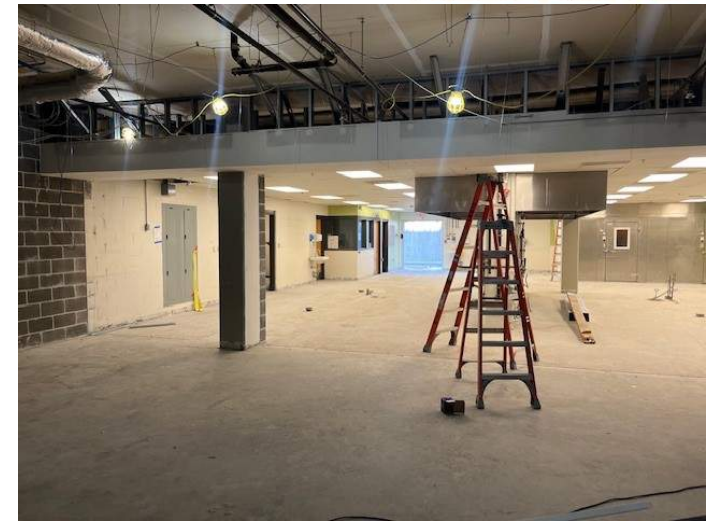
Kitchen Build Back
