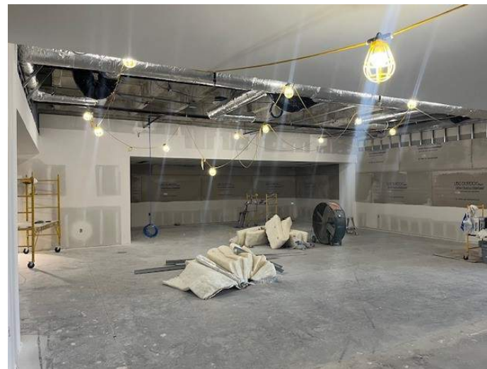
New Seating Area Progress
