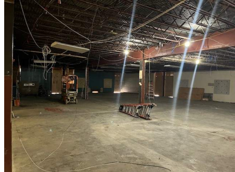
1964 (Area A) Progress
