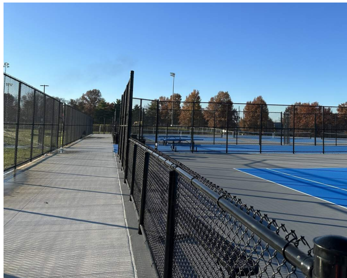
East Concourse Looking South
