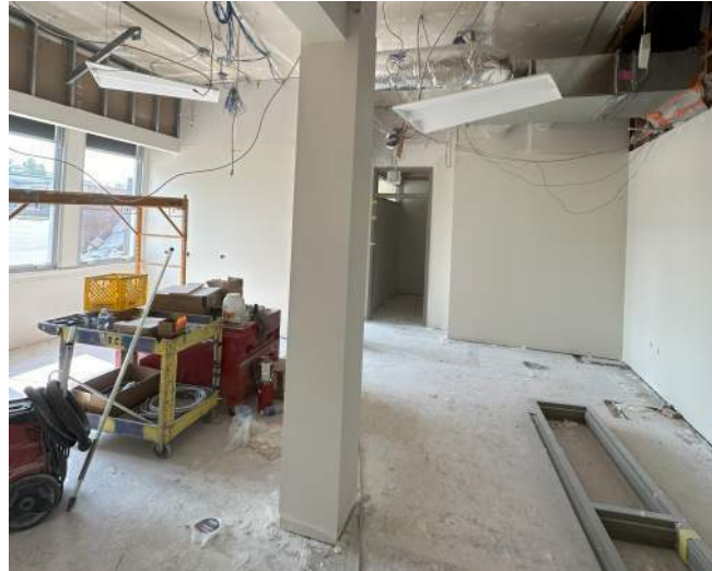
Franklin - Main Office
