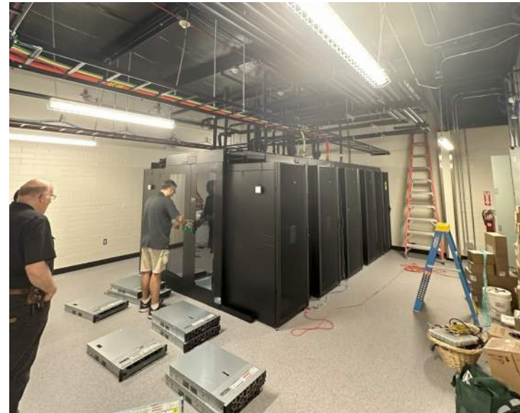
Data Pod Install
