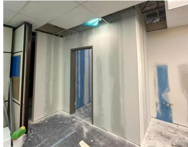
Doniphan - SPED Restroom Remodel
