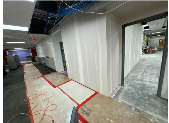
EPiC Elementary - Interior Renovation
