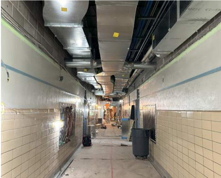
Ridgeview - Corridor MEP Install
