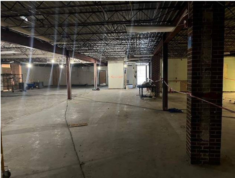
1964 (Area A) Progress
