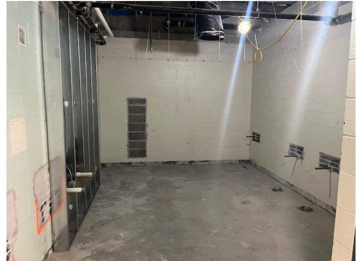
Bathroom Build Back
