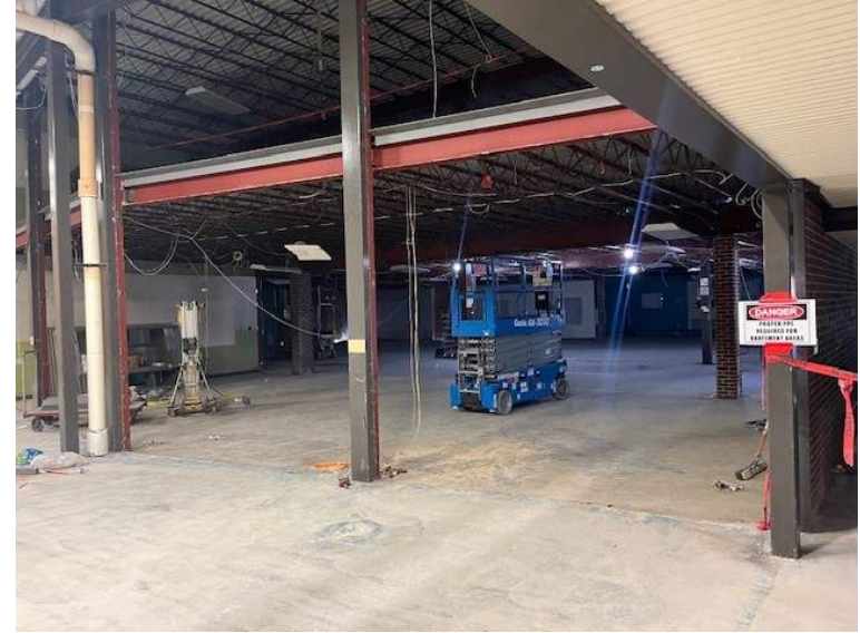
1964 (Area A) Progress
