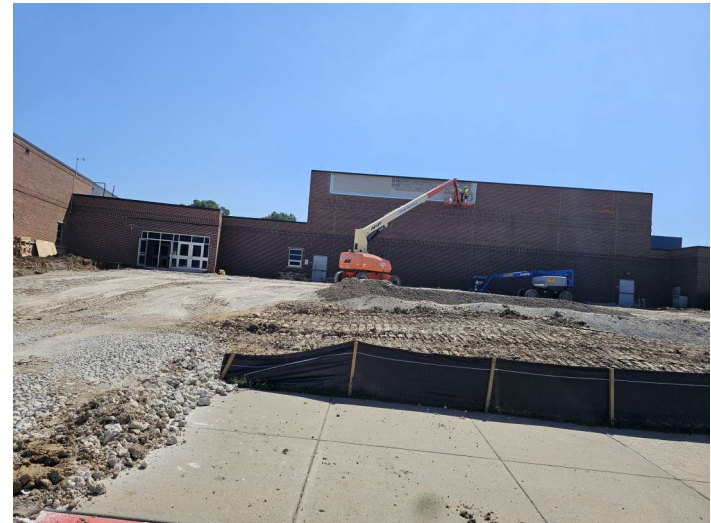
DMS - Building Pad
