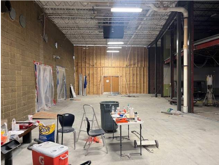
1964 (Area A) Progress
