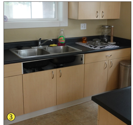
Kitchen sink cabinet face trim panel is missing. The kitchenette used by the community.
