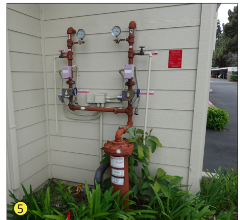
Fire sprinkler system provided at each building.
