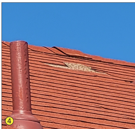
4 Missing one single at right wing of building 3459.
