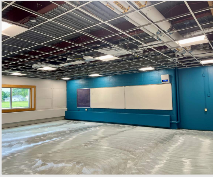
Top Left: classroom floor prepped with adhesive to receive new flooring at Kegonsa Elementary following paint and ceiling grid install
