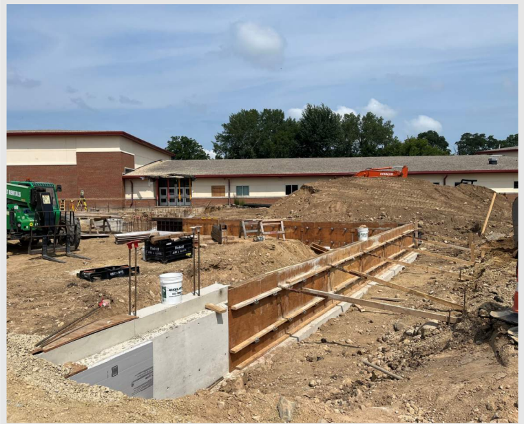
Bottom Right: a view of the progress at River Bluff as the last stretch of foundation walls are formed up and ready to pour
