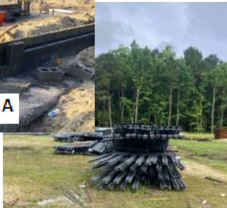
STEEL FOR VERTICAL CONSTRUCTION
