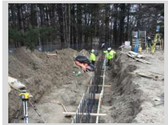
Wall Footing Formwork at Exterior Wall
