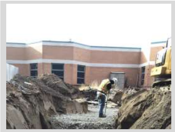
Excavation and Compaction Testing for Wall Footing
