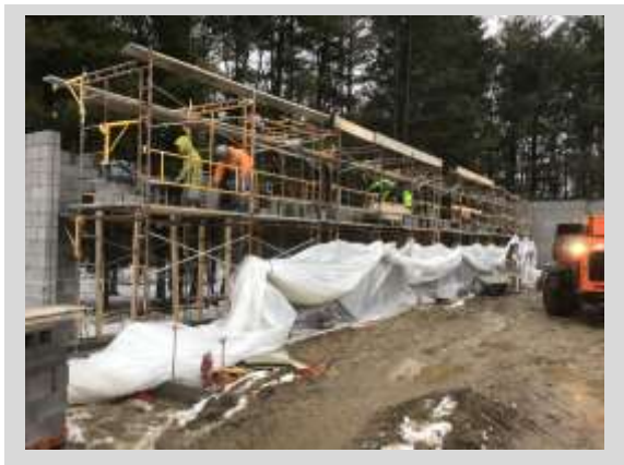
CMU Block Placement at North Wall
