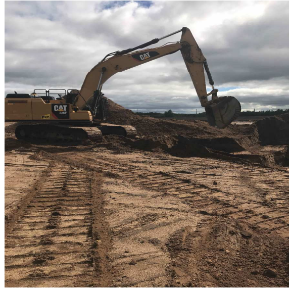
Area 1 – Learning Neighborhood footing excavation
