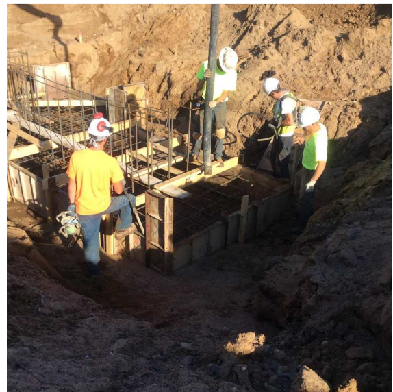
Area 1 – Learning Neighborhood concrete
