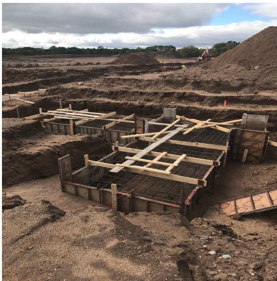
Area 1 – Learning Neighborhood concrete forms
