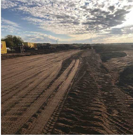
Gravel access road at west entrance
