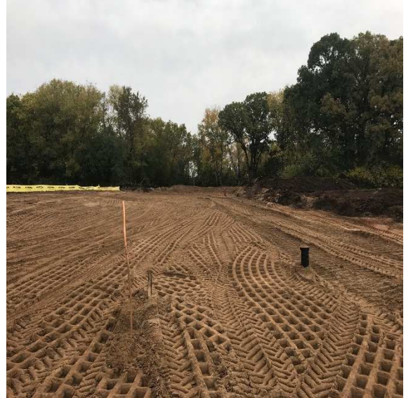
North Access Road subgrade & utilities
