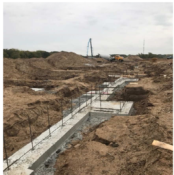
Area 1 – Learning Neighborhood footings
