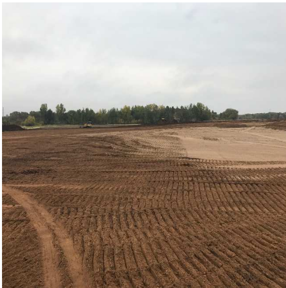
Athletic Complex Grading
