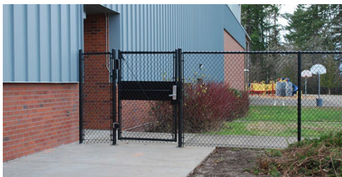
Fencing project with locks to prevent entry at Rosedale Elementary
