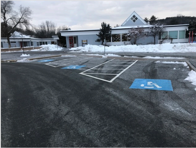
OVERVIEW OF ACCESSIBLE PARKING AREA
