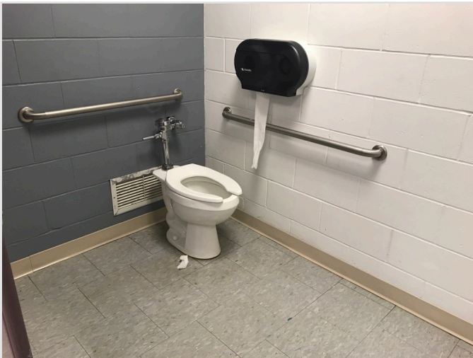
TOILET STALL OVERVIEW
