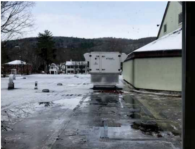
21 - ENERGY RECOVERY VENTILATOR
