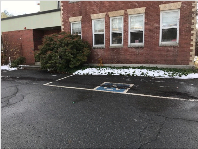
OVERVIEW OF ACCESSIBLE PARKING AREA
