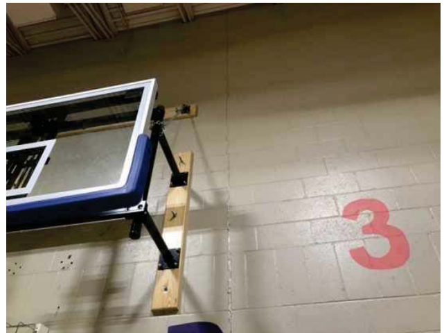
34 - INTERIOR WALL CRACKING - SEAL
