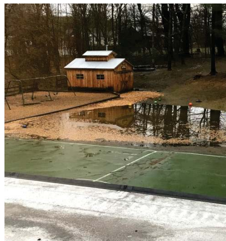
36 - SITE PONDING - REPAIR
