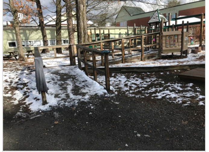
ACCESSIBLE ROUTE TO PLAYGROUND
