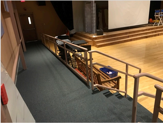
ACCESSIBLE INTERIOR RAMP
