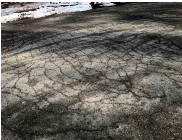
35 - ALLIGATOR CRACKING - REPAIR
