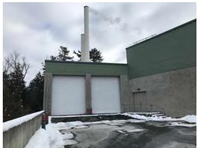
6 - CENTRAL HEATING PLANT
