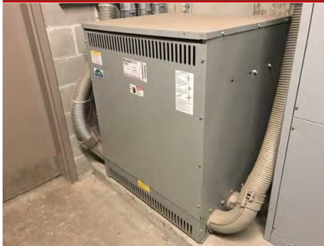
25 - SECONDARY TRANSFORMER
