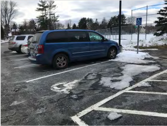
OVERVIEW OF ACCESSIBLE PARKING AREA
