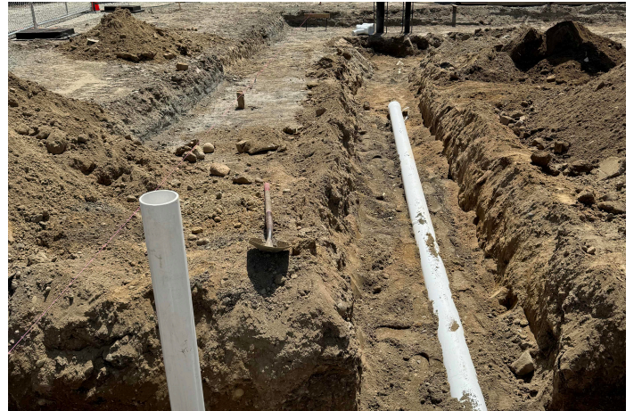
Underground sanitary drainage installation
