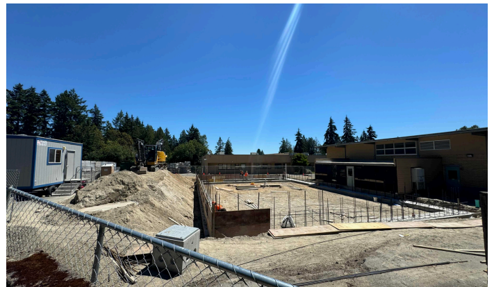
Erection of forms for stem walls
