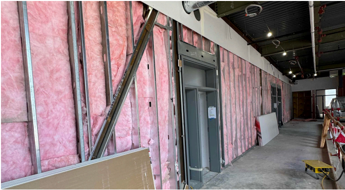
Insulation install
