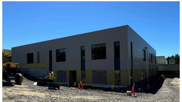
June Construction Progress
