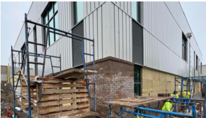
Brick & Metal siding installation
