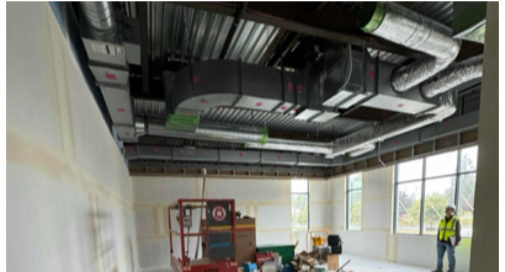
Duct Work & Drywall Installation, Mud & Tape Progression
