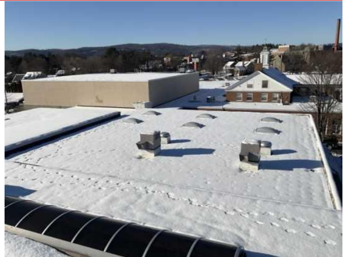
14 - OVERVIEW OF ROOFS
