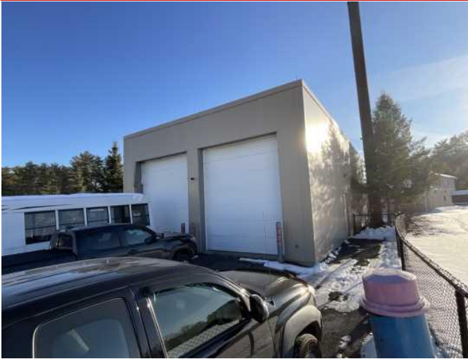
7 - WOOD CHIP PLANT
