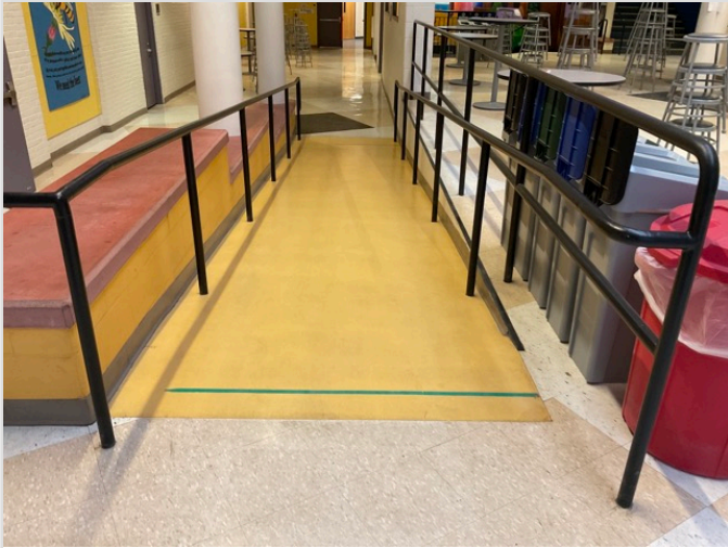
ACCESSIBLE INTERIOR RAMP
