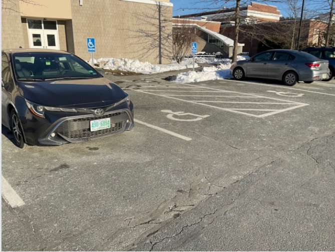
OVERVIEW OF ACCESSIBLE PARKING AREA
