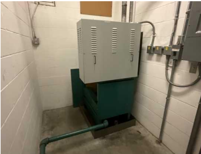
39 - ELEVATOR MACHINERY
