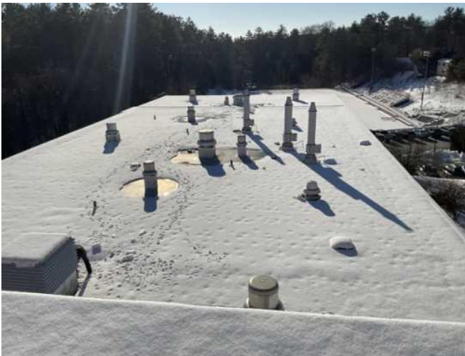
15 - OVERVIEW OF ROOFS
