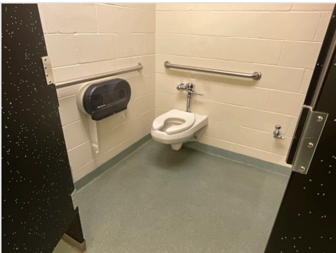
TOILET STALL OVERVIEW
