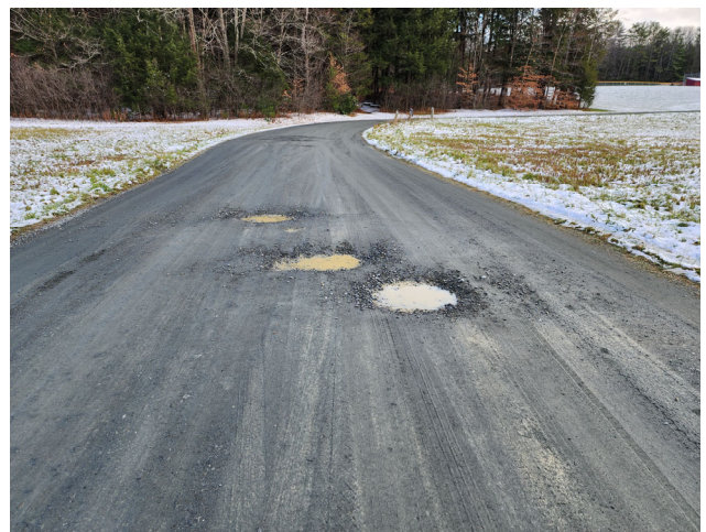
12 - DRIVEWAY POTHOLES - REPAIR
