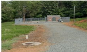
The town's Elizabeth Brady Pumping station. The new station would be similarly configured.
