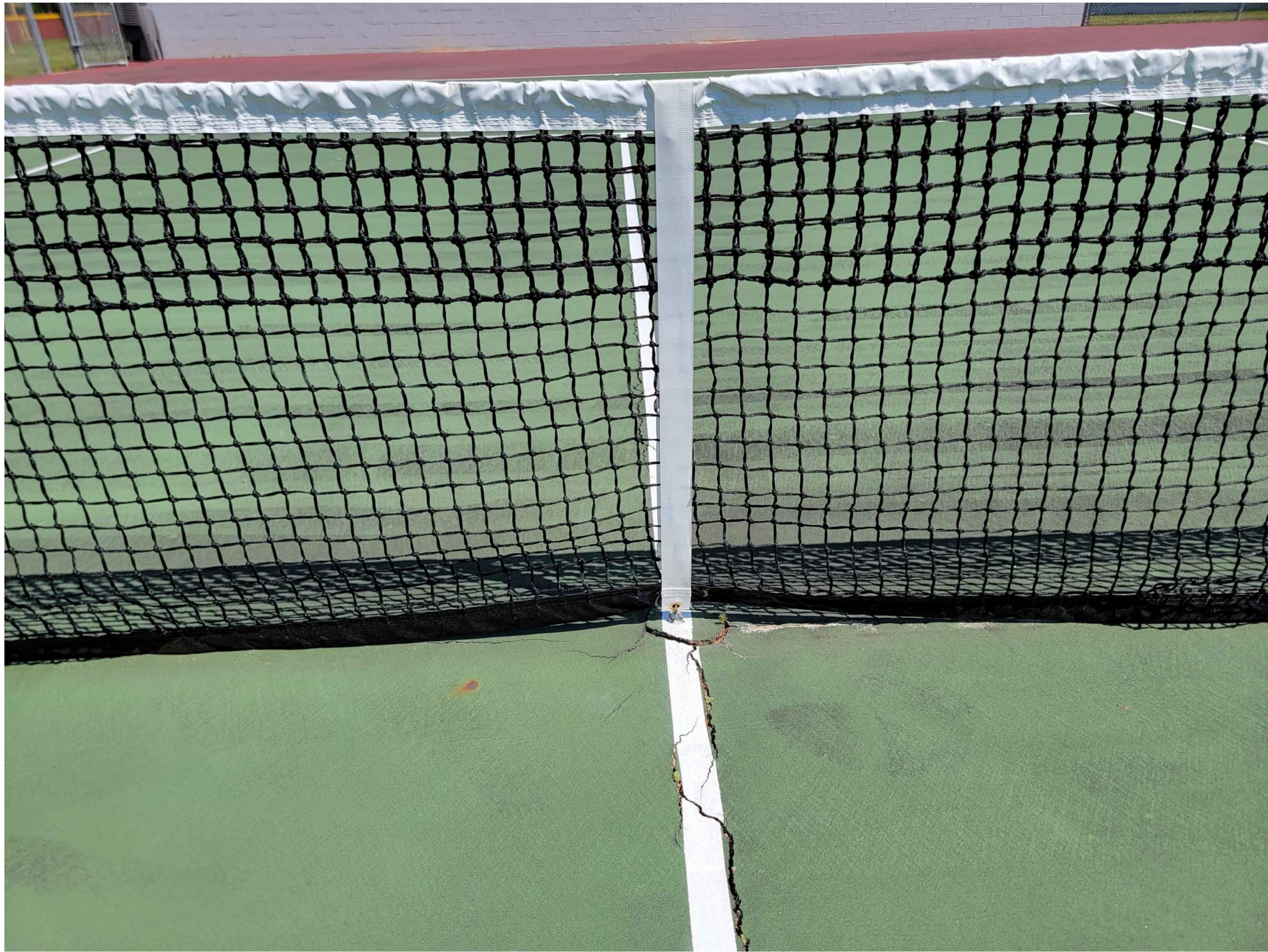
MINOR CRACKS ALONG NET ANCHOR STRAP
