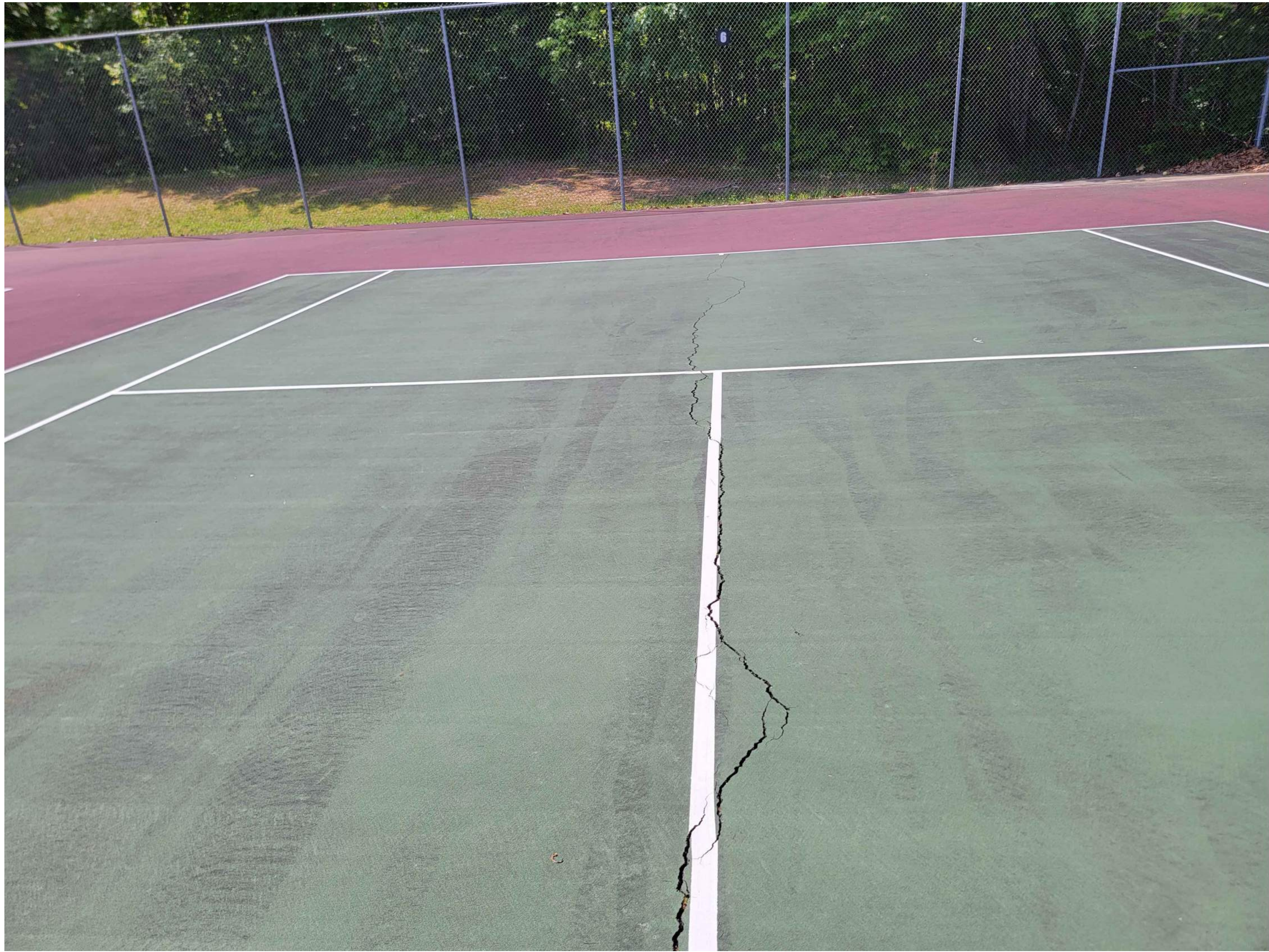
MINOR CRACKS
