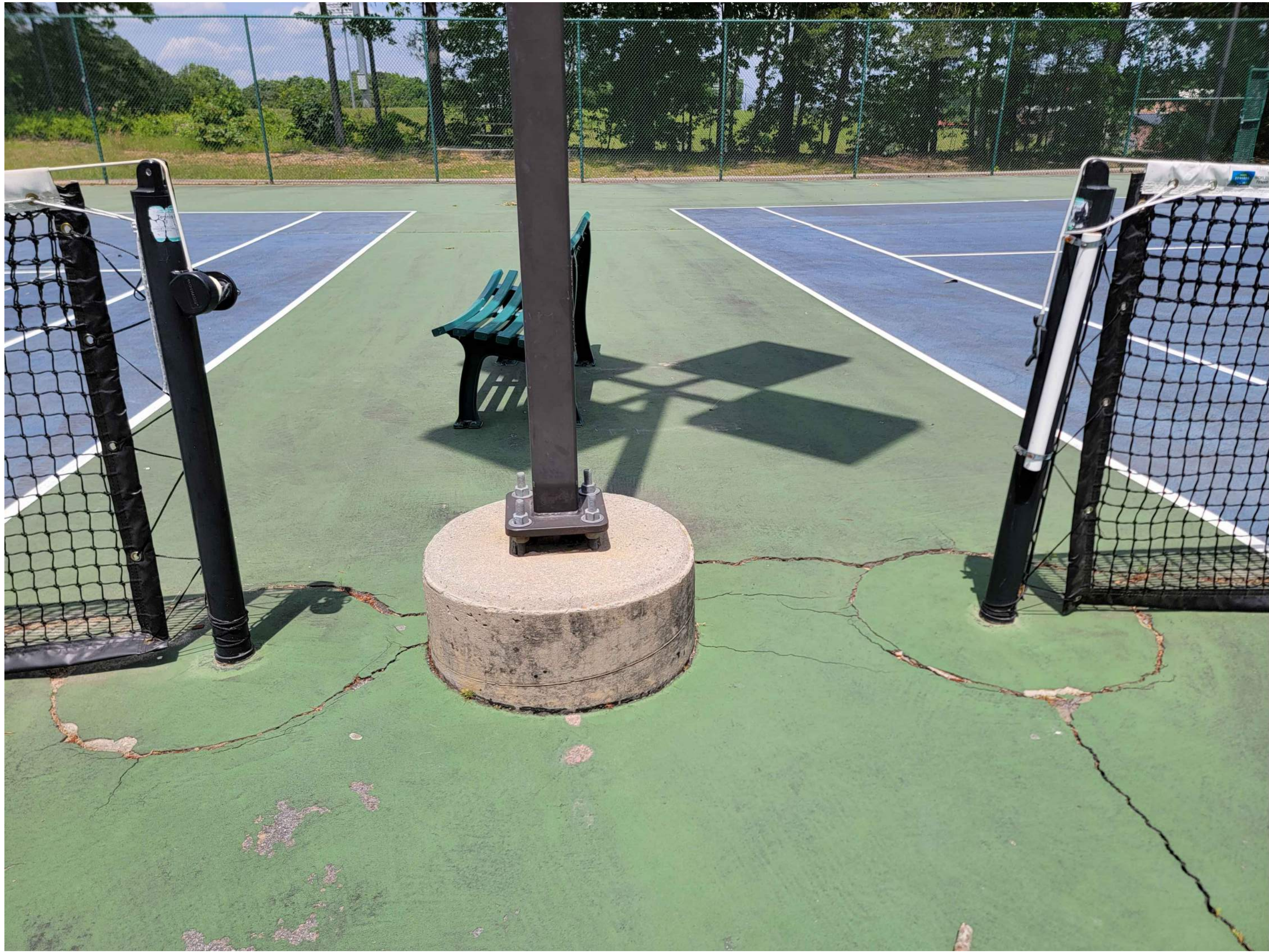
MINOR CRACKS ALONG NET POST FOOTING
