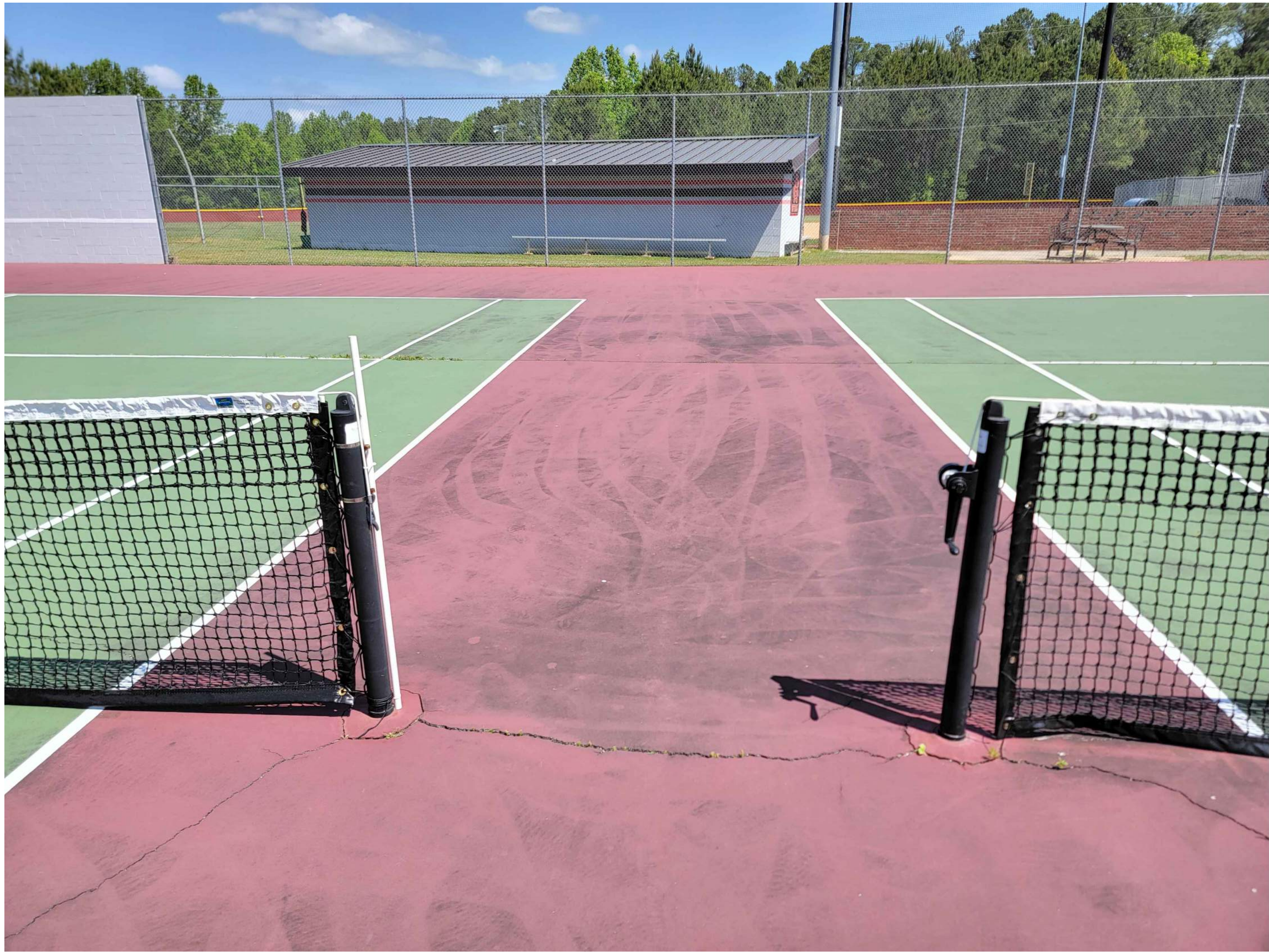
MINOR CRACKS ALONG NET POST FOOTING
