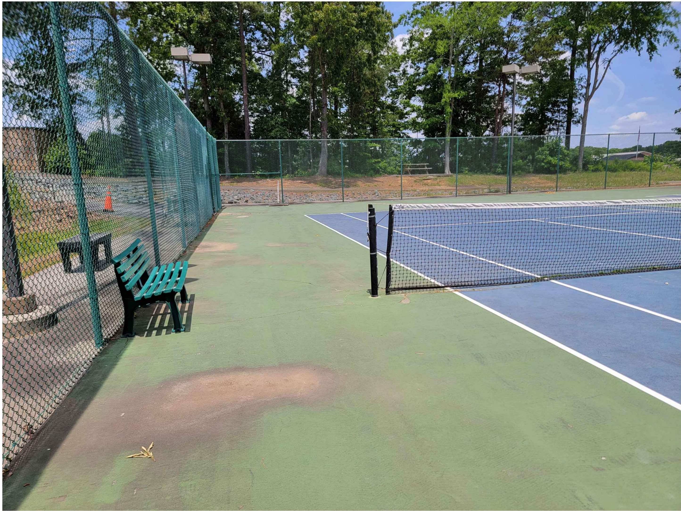
LOW SPOT TO BE PATCHED AND LEVELED
