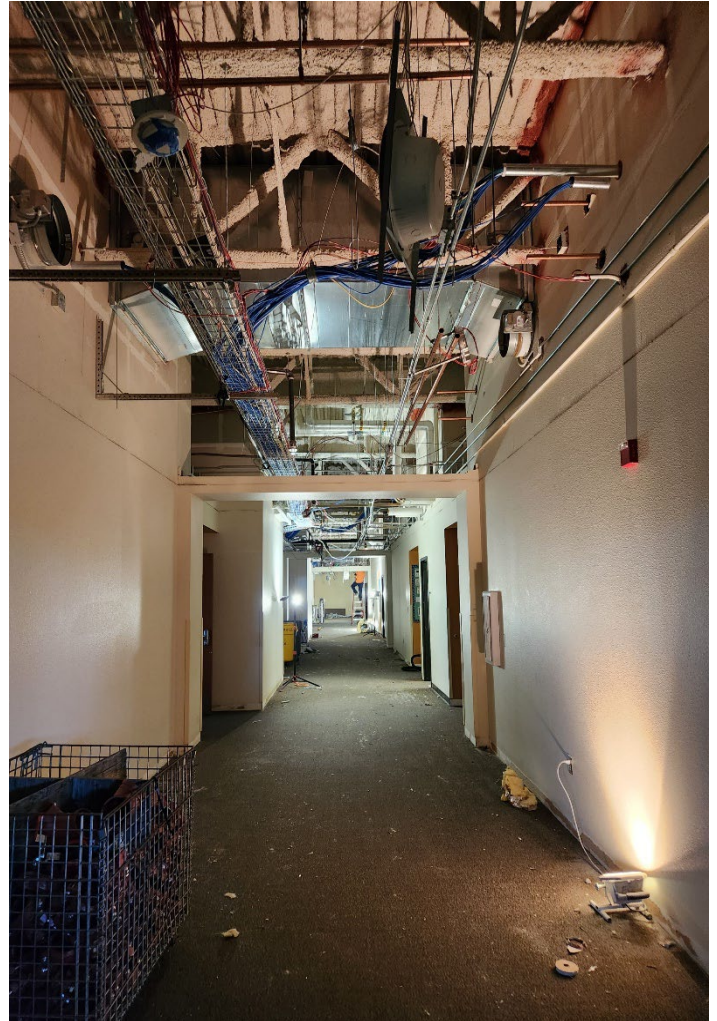
LOHS Science Hallway Ceiling Demolition
