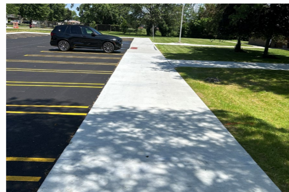
New sidewalk, paving, & striping
