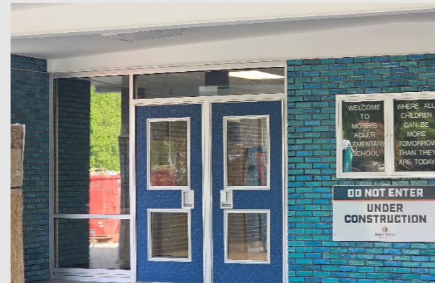
New exterior doors and glazing
