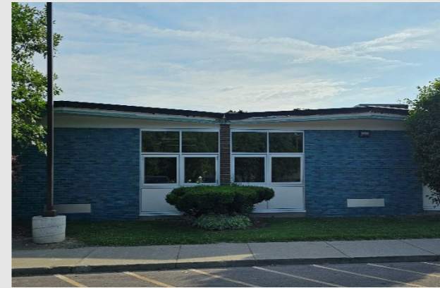
New exterior glazing
