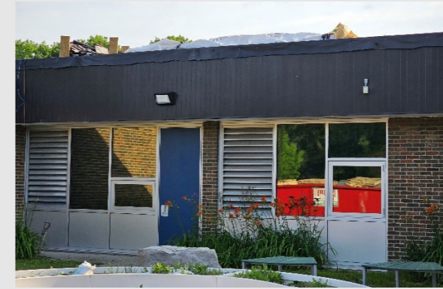
New exterior glazing, louvers, & doors
