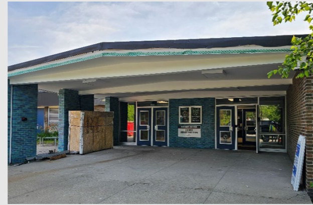
Main entry canopy soffit replacement
