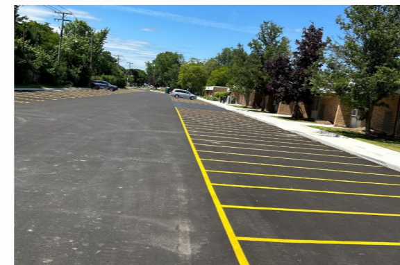
New sidewalk, paving, & striping
