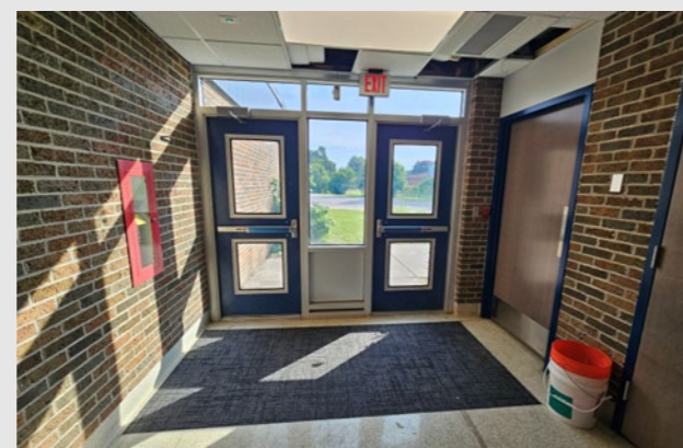
New exterior doors and glazing
