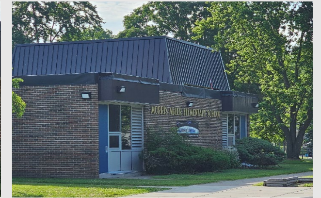
New metal panel, glazing, louvers, & doors
