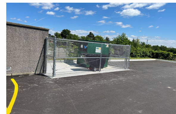
New paving & fencing
