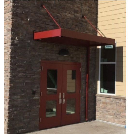
Canopy at Exterior Doors
