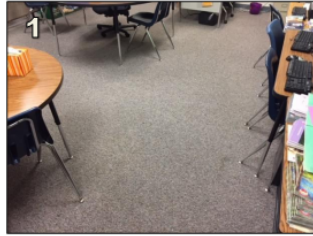
1 Rolled carpet throughout classrooms is stained, in poor condition and should be replaced.
