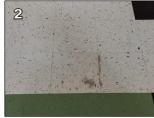
2 Conditions of VCT throughout corridors and various classrooms varies; as replacing in patches would likely appear worse, replacement is recommended.
