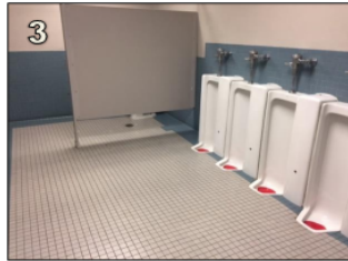
3 Original floor mounted urinals should be replaced.
