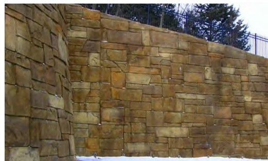
Figure 6-2: Shotcrete Sculpted Facing Example Photo
