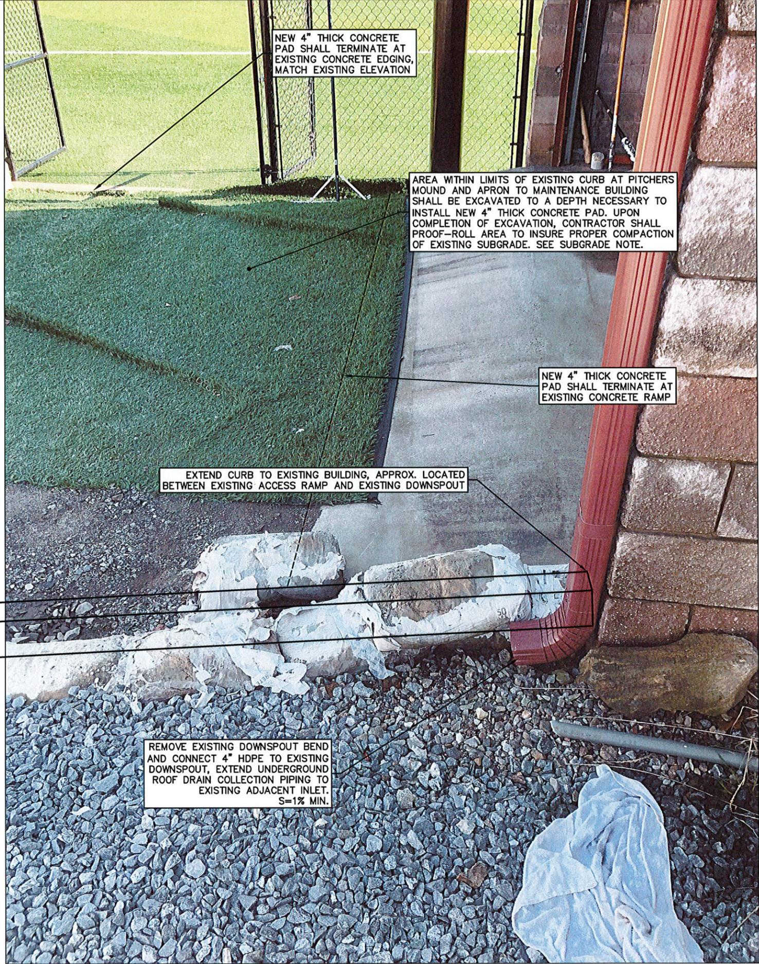
NEW 4" THICK CONCRETE PAD SHALL TERMINATE AT EXISTING CONCRETE EDGING, MATCH EXISTING ELEVATION
