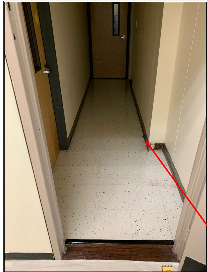
Photos 32 & 33 Damaged VAT in the Hallway in Room 209
