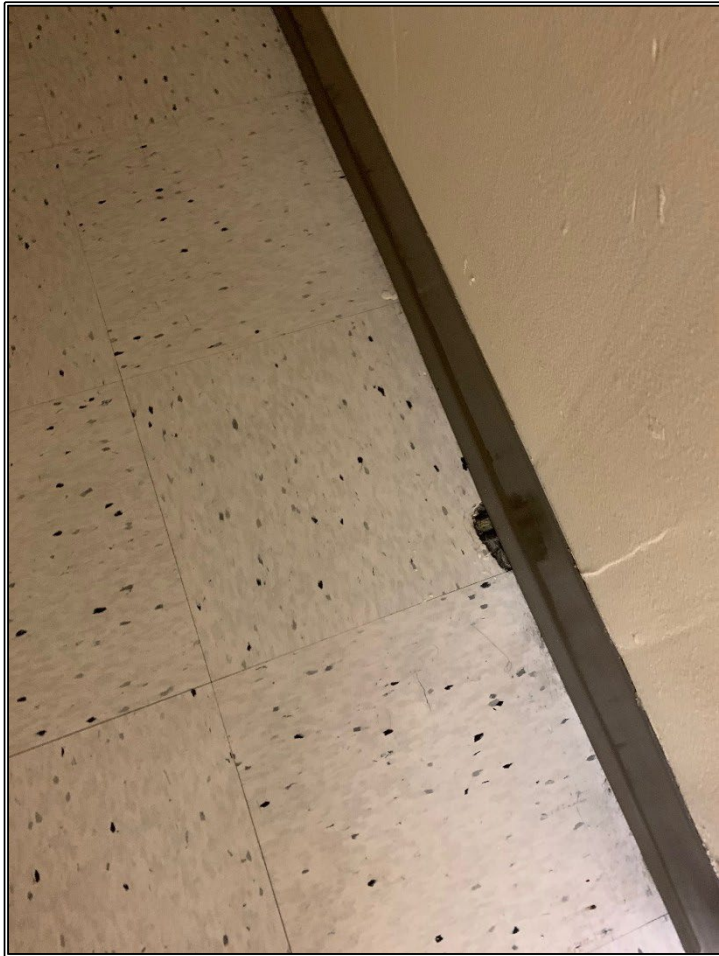
Photos 32 & 33 Damaged VAT in the Hallway in Room 209
