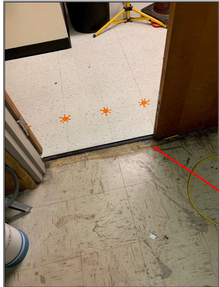
Photos 38 & 39 Damaged VAT in the Basement Electrical Closet
