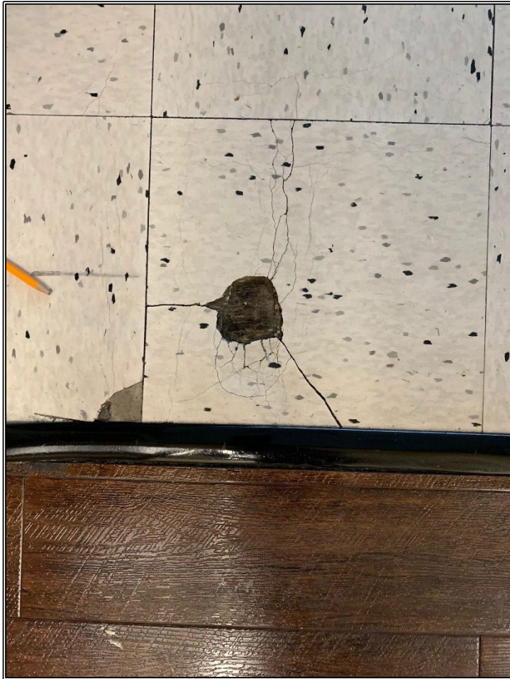
Photos 6 & 7 Damaged VAT in Classroom 106
