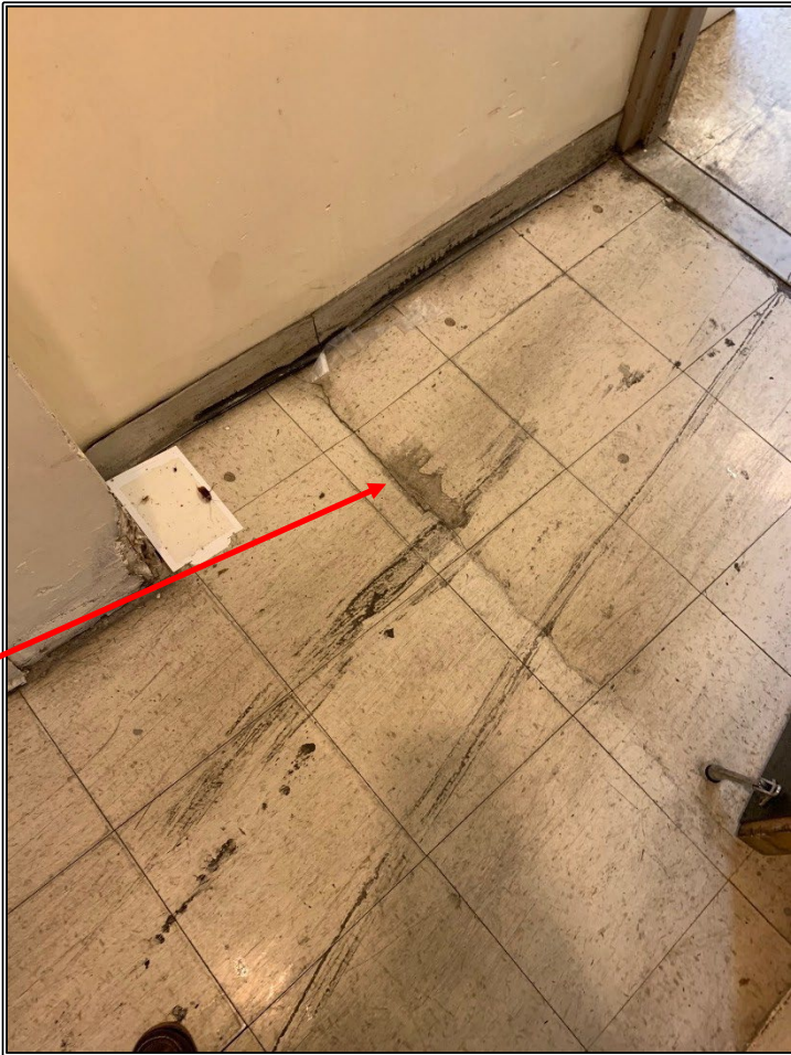
Photos 13 & 14 Damaged VAT in the Hallway to Exit behind Kitchen
