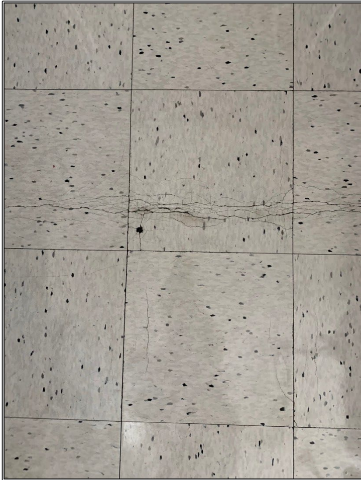
Photos 30 & 31 Damaged VAT in Classroom 207
