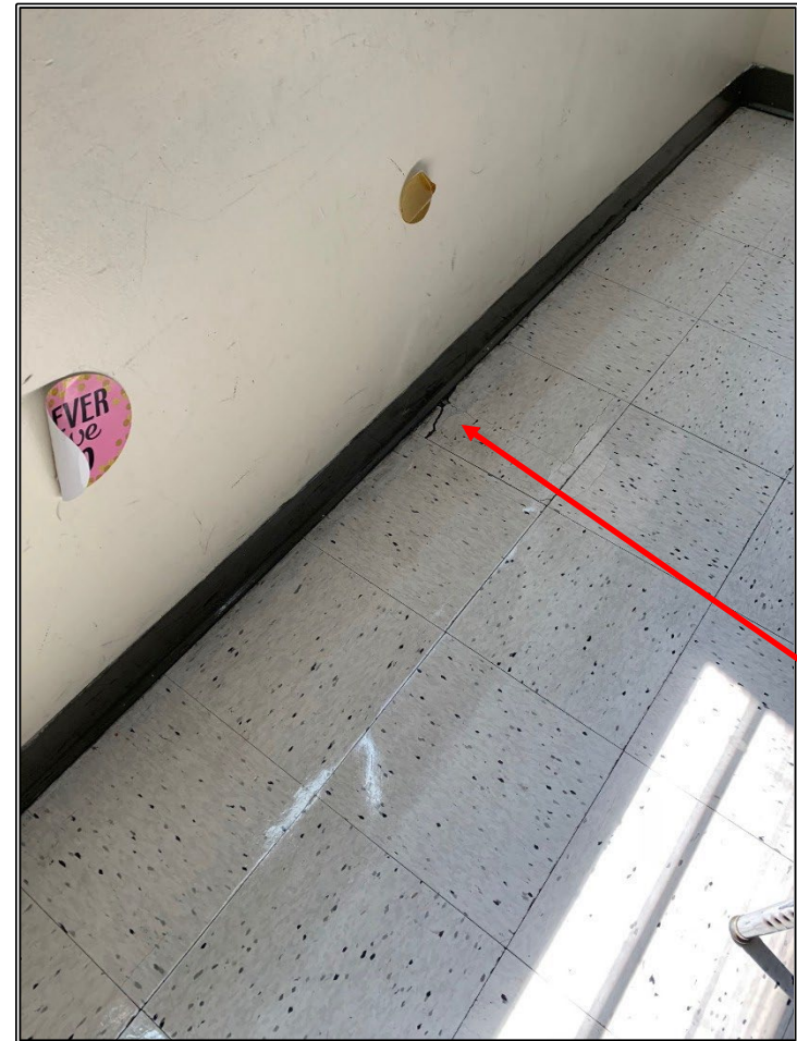
Photos 28 & 29 Damaged VAT in Classroom 207
