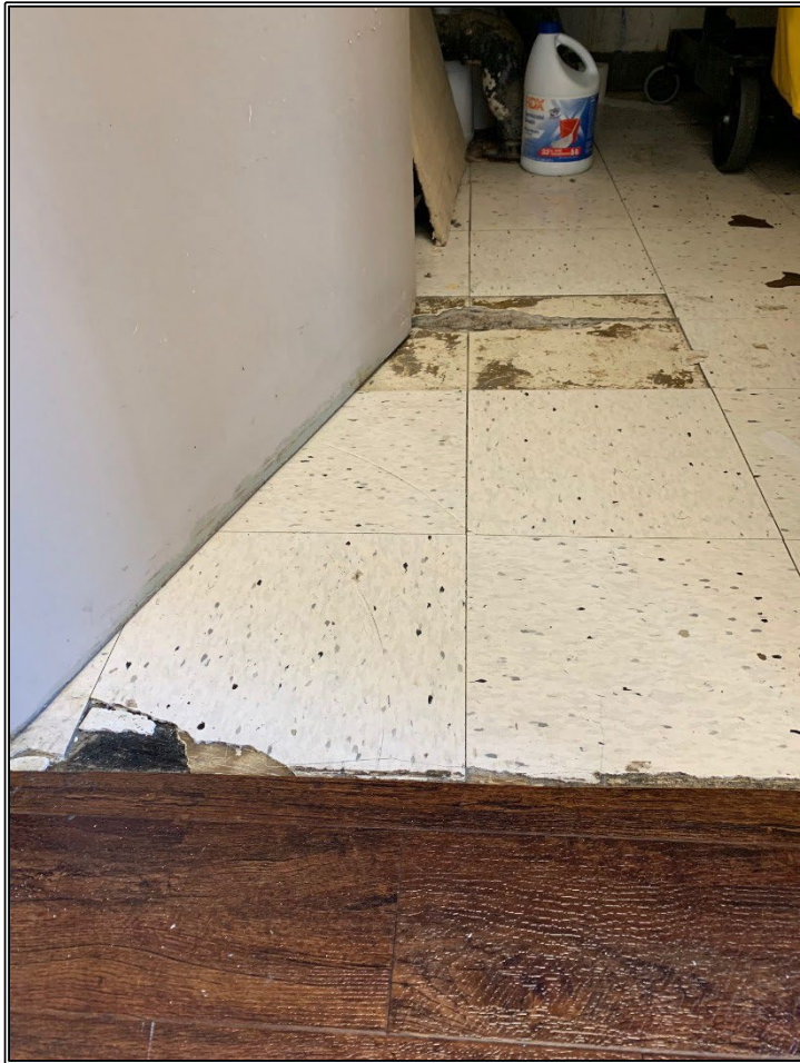
Photos 34 & 35 Damaged VAT in the Custodial Closet adjacent to Classroom 208
