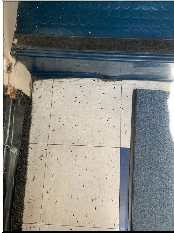
Photos 17-19 Damaged VAT in the Center Stairwell by Main Entrance (1 st Floor)
