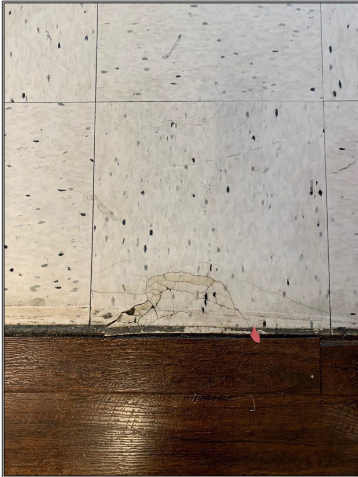
Photos 26 & 27 Damaged VAT in Classroom 205
