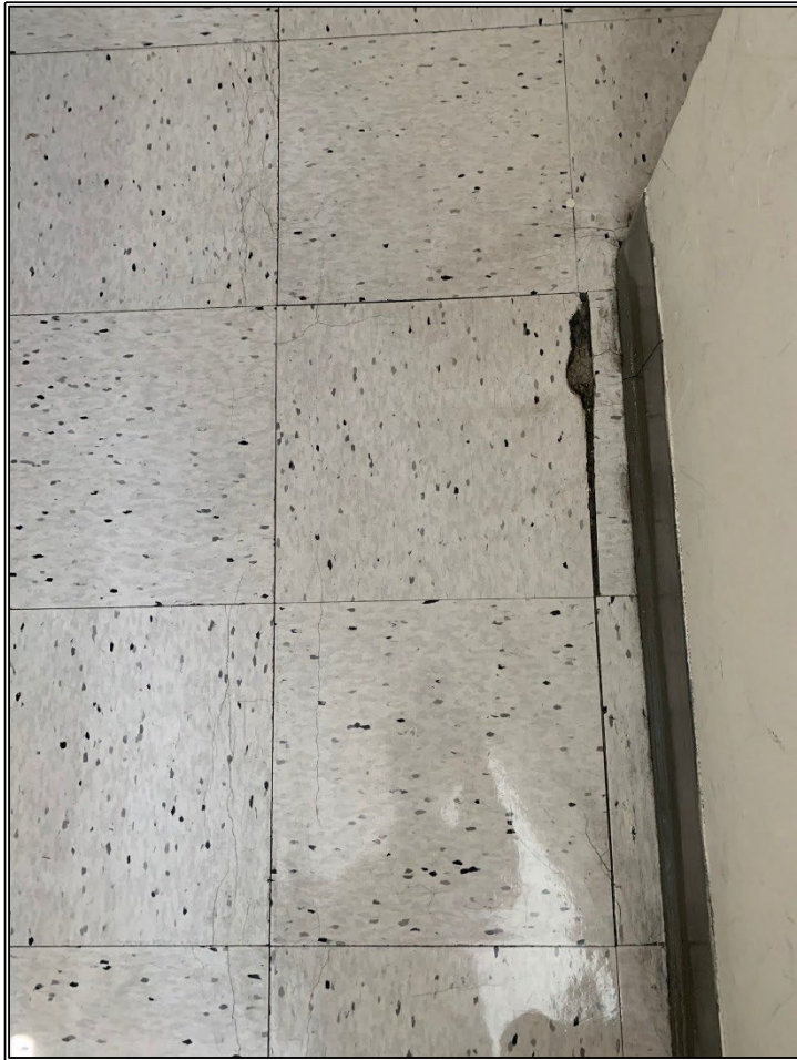
Photos 28 & 29 Damaged VAT in Classroom 207
