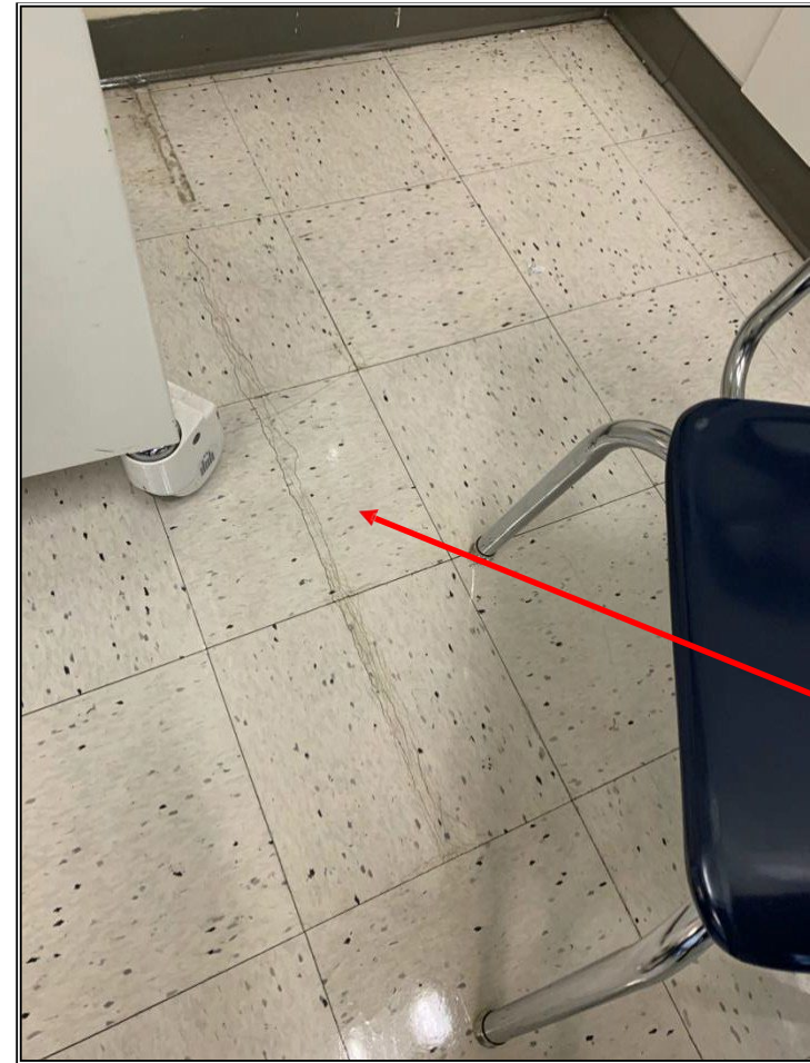
Photos 44 & 45 Damaged Floor Tile in Classroom 204
