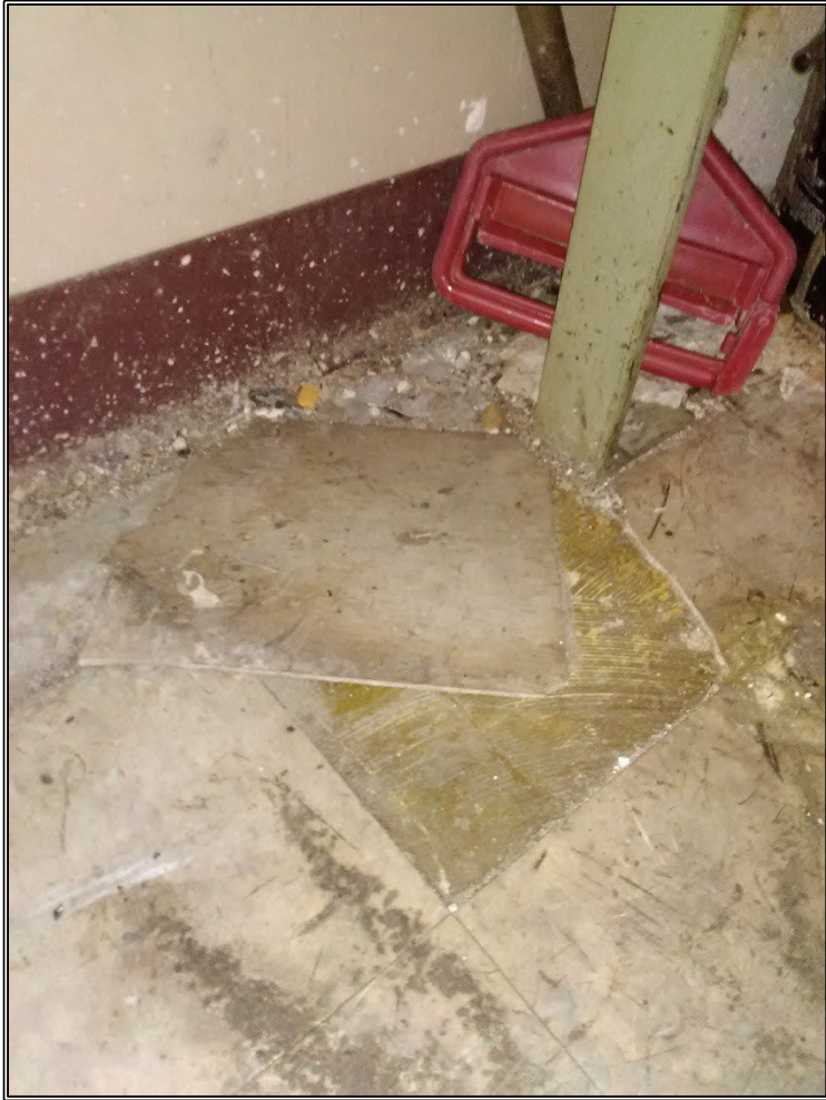
Photos 40 & 41 Damaged VAT at the Roof Access
