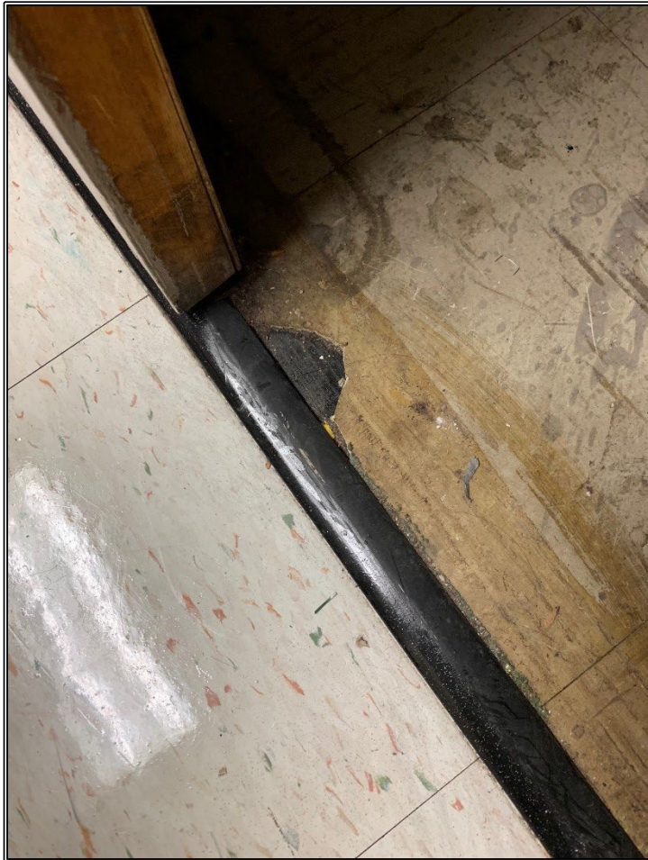
Photos 38 & 39 Damaged VAT in the Basement Electrical Closet
