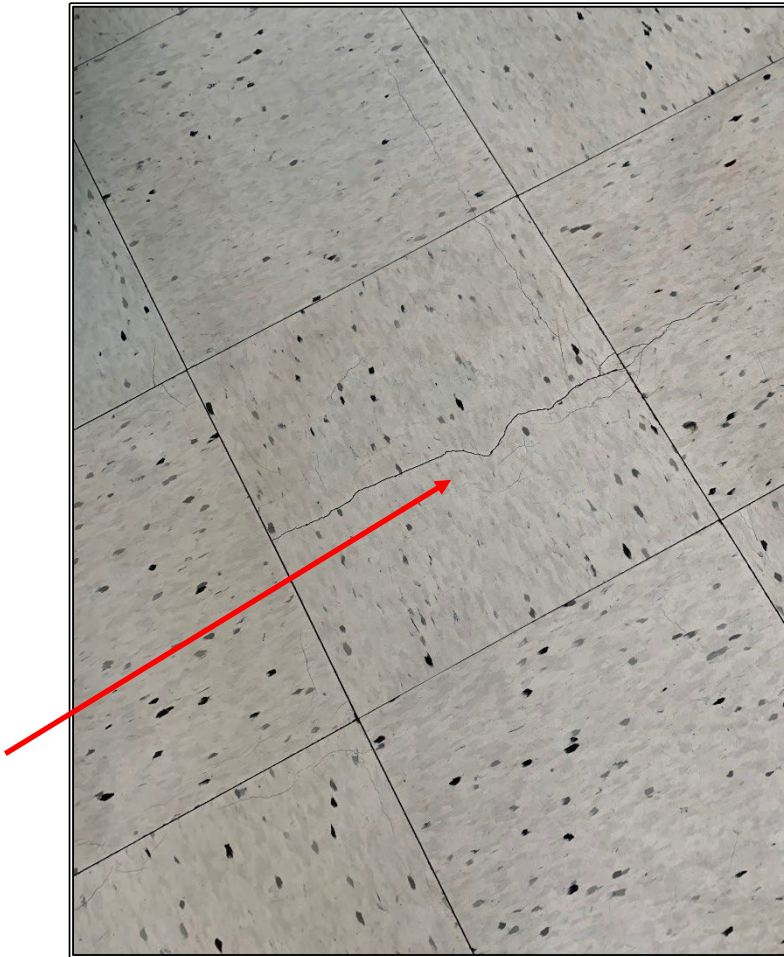
Photos 8 & 9 Damaged VAT in Classroom 107
