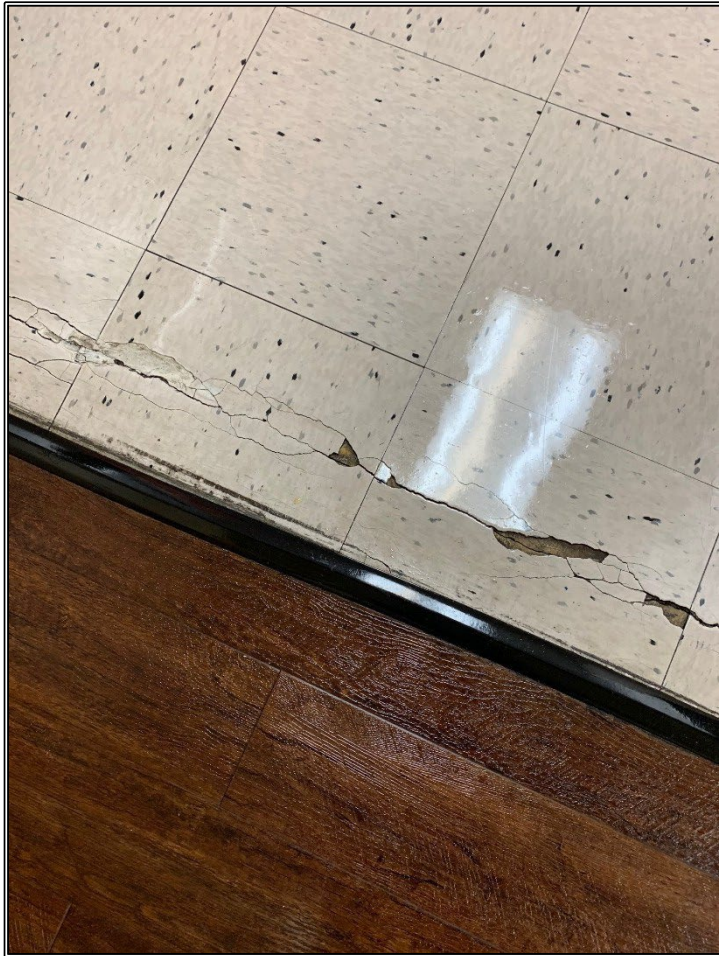
Photos 36 & 37 Damaged VAT in the North Stairwell by Elevator (2 nd Floor)
