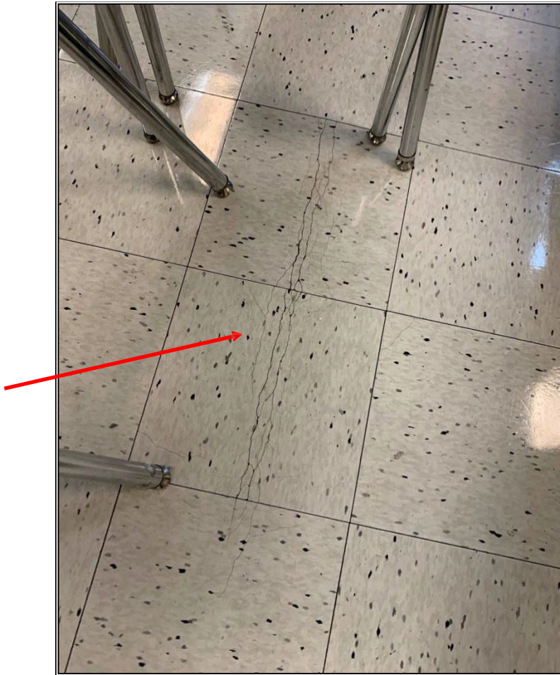
Photos 44 & 45 Damaged Floor Tile in Classroom 204
