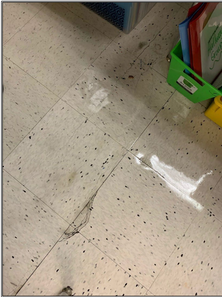
Photos 4 & 5 Damaged VAT in Classroom 102
