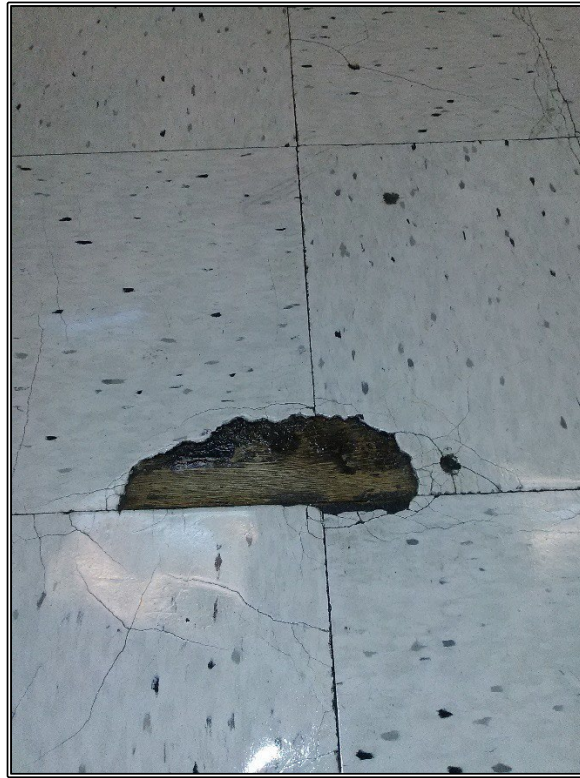
Photos 20-22 Damaged VAT in Classroom 201
