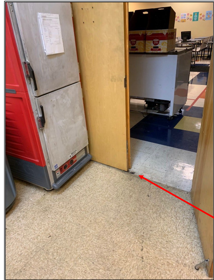
Photos 15 & 16 Damaged VAT in the Cafeteria
