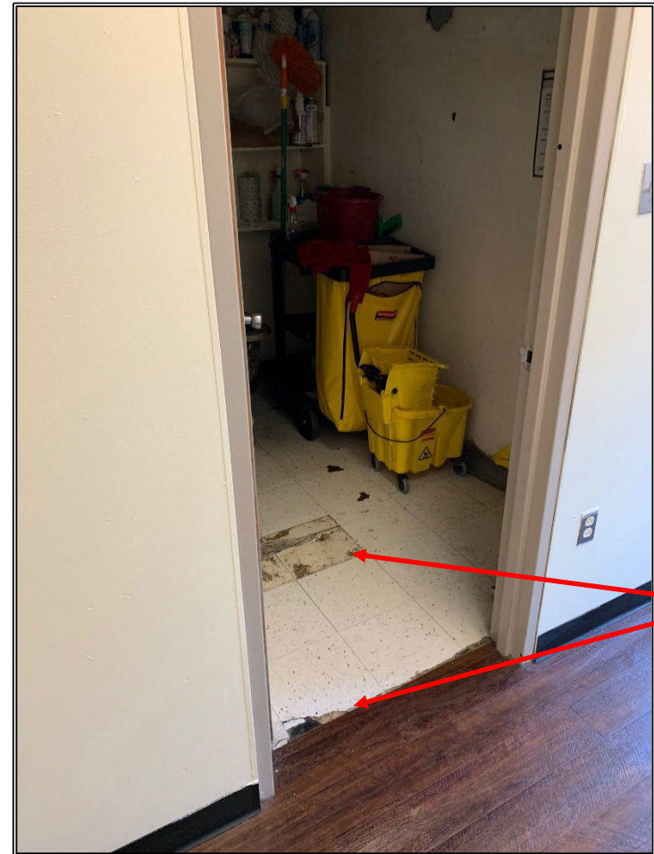
Photos 34 & 35 Damaged VAT in the Custodial Closet adjacent to Classroom 208
