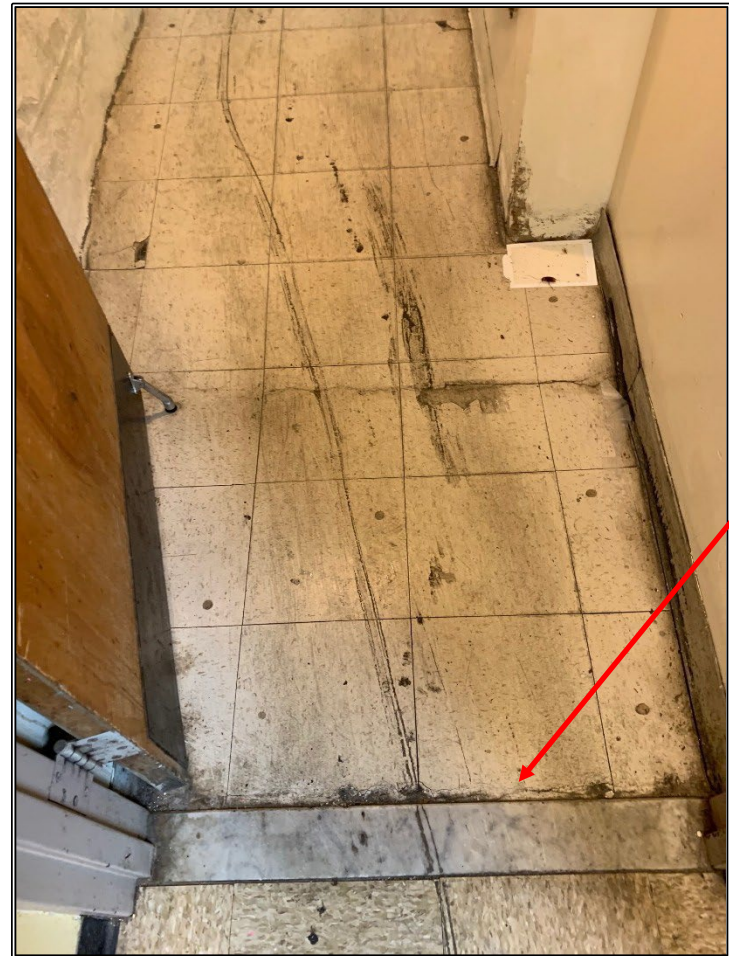
Photos 13 & 14 Damaged VAT in the Hallway to Exit behind Kitchen
