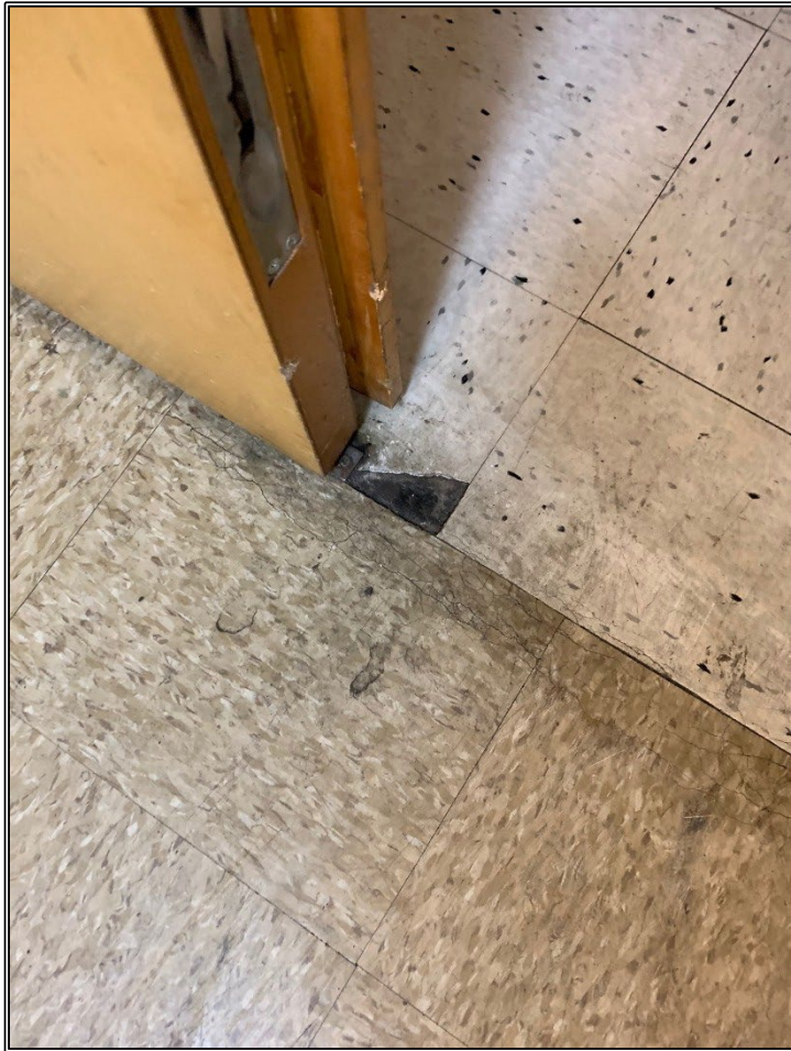
Photos 15 & 16 Damaged VAT in the Cafeteria
