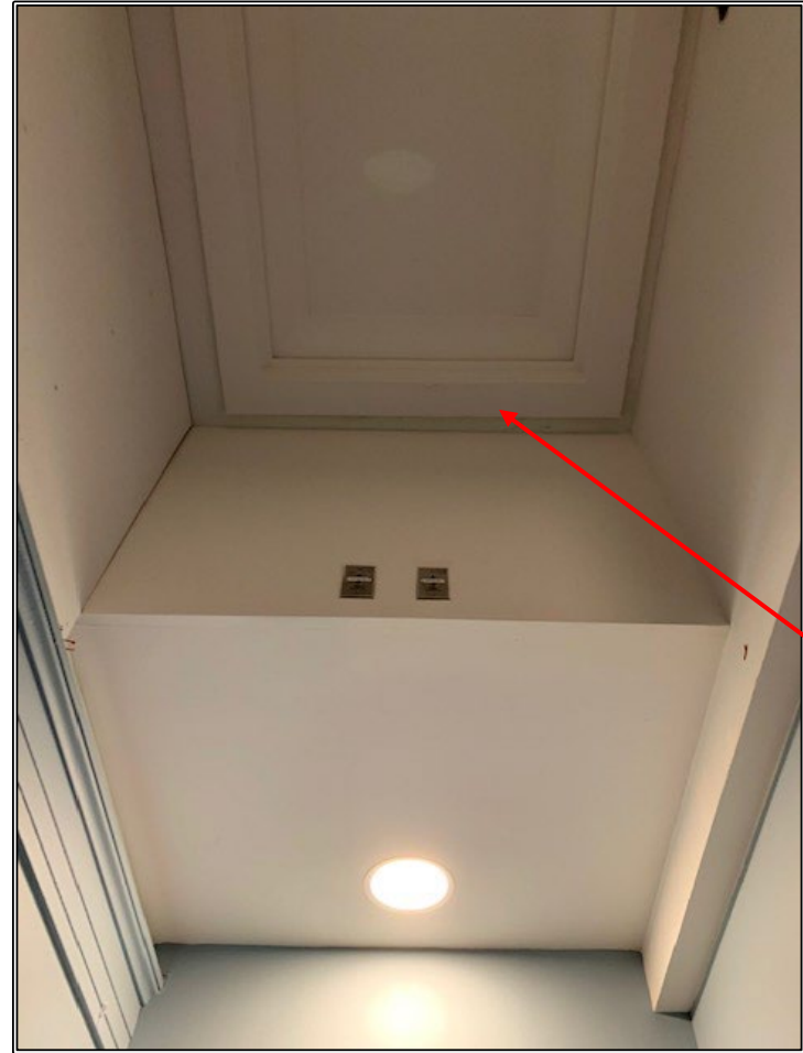
Photos 5 & 6 Flaking Paint applied to the Ceiling in the 2 nd Floor Hallway outside of the Science Room
