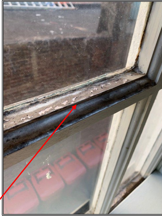
Photos 19-21 Damaged Paint associated with Window Sash and Missing Windowpane
