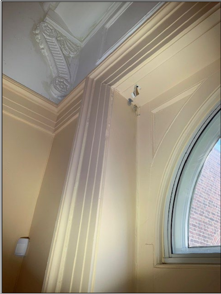
Photos 7 & 8 Cracking Paint associated with Window Frames in Room 205
