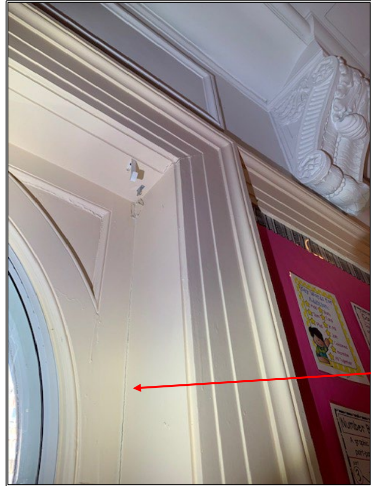
Photos 7 & 8 Cracking Paint associated with Window Frames in Room 205
