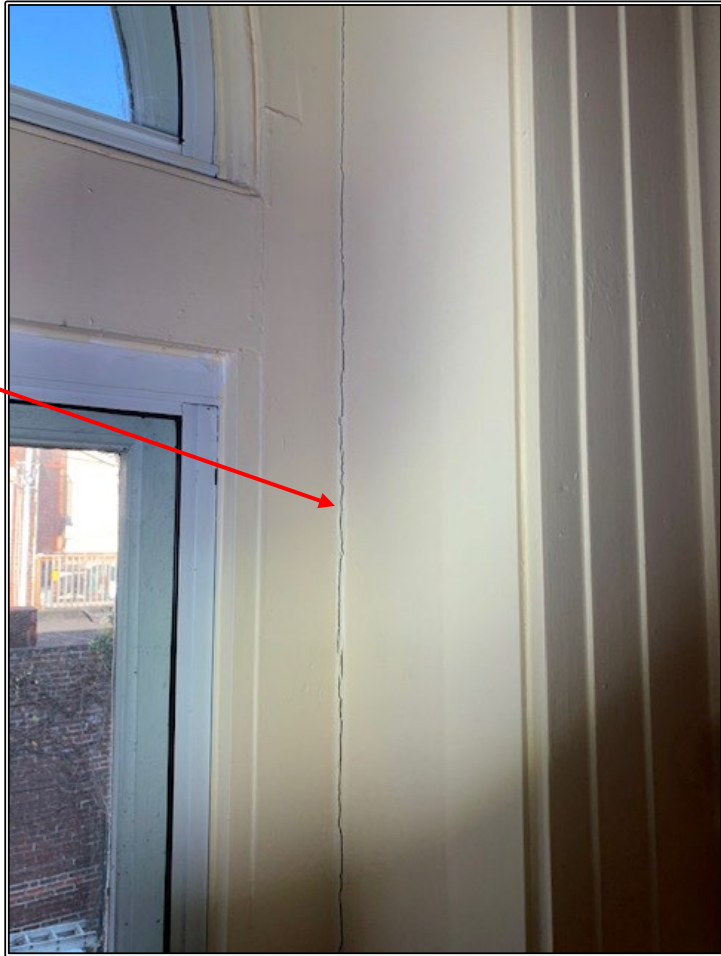
Photos 9 & 10 Cracking Paint associated with Window Frames in Room 205
