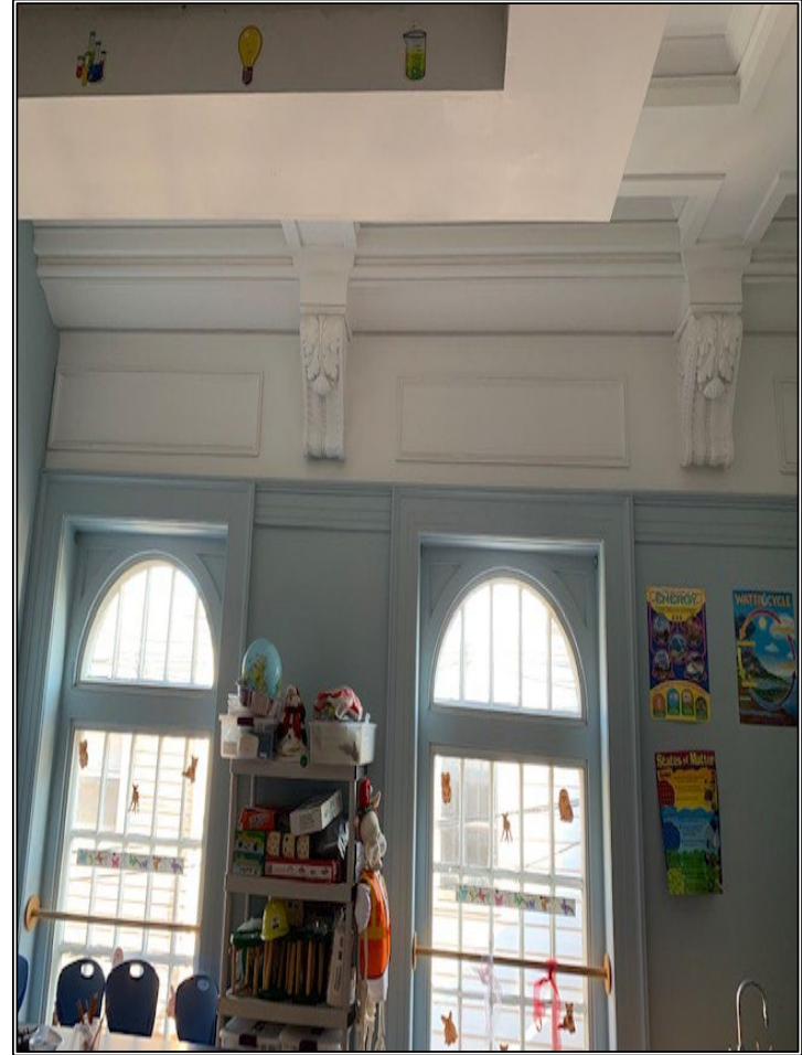
Photos 3 & 4 Flaking Paint applied to Decorative Ceiling Plaster in the Science Room
