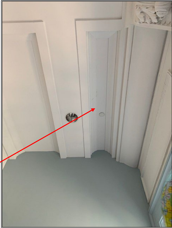
Photos 3 & 4 Flaking Paint applied to Decorative Ceiling Plaster in the Science Room
