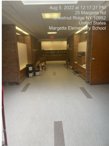
Margetts ES – Flooring Replacement Work – Progress Photos: New Flooring & Base – Installations
