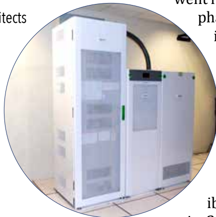
Housing for the data center's new UPS
