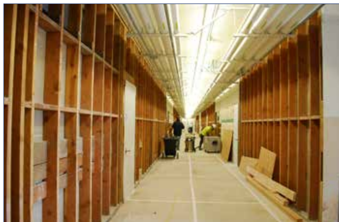
BEFORE: hallway walls stripped for seismic and other improvements
