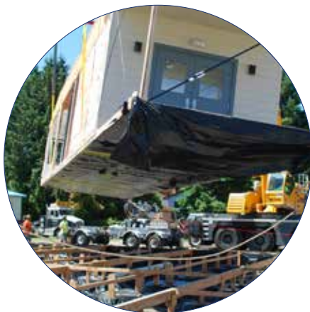
Modular section being installed on foundation
