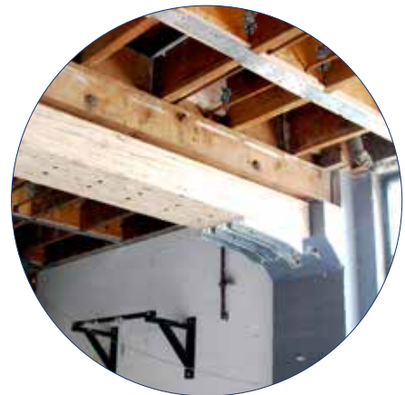
Seismic bracing was added throughout the Peter Boscow building
