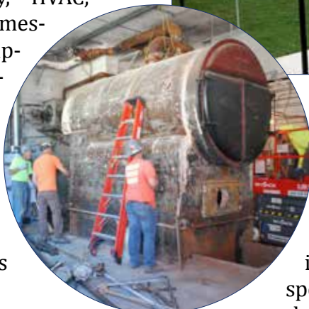
Old boiler being removed
