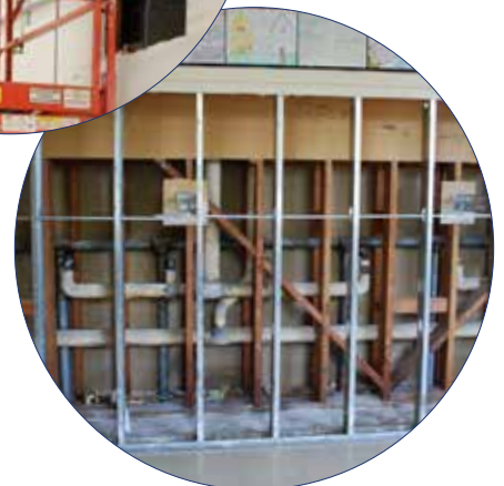
Plumbing upgrades in progress
