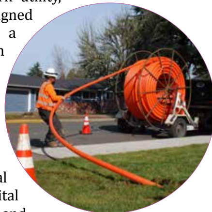
Undergrounding conduit for dark fiber installation
