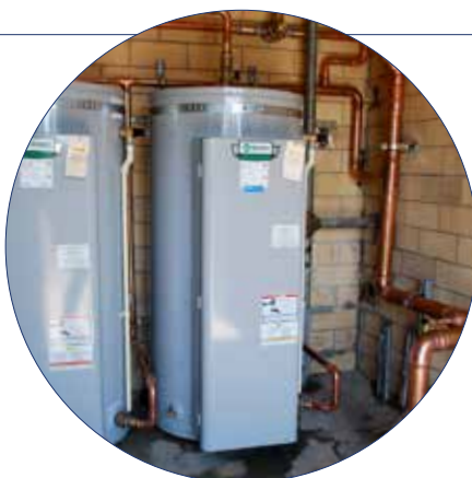
New water heaters and plumbing replaced the old boiler system at Hare Field
