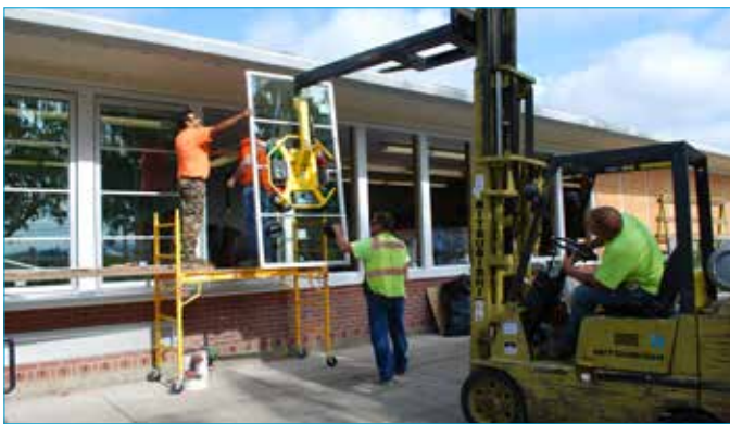
Contractors install new windows at Groner Elementary
