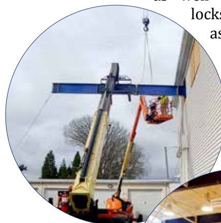
Installing new roof trusses in gym
