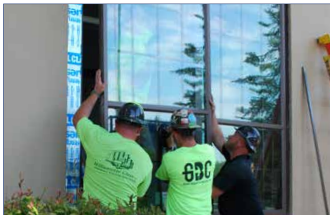
Installation of double-paned windows
