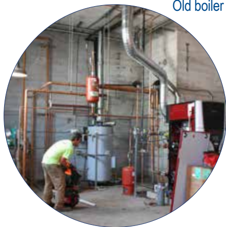
A new water heater, pipes and HVAC equipment in the old boiler's space
