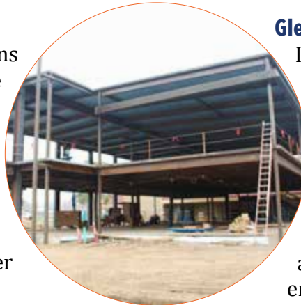
Steel construction of Glencoe's new media center/classroom wing
