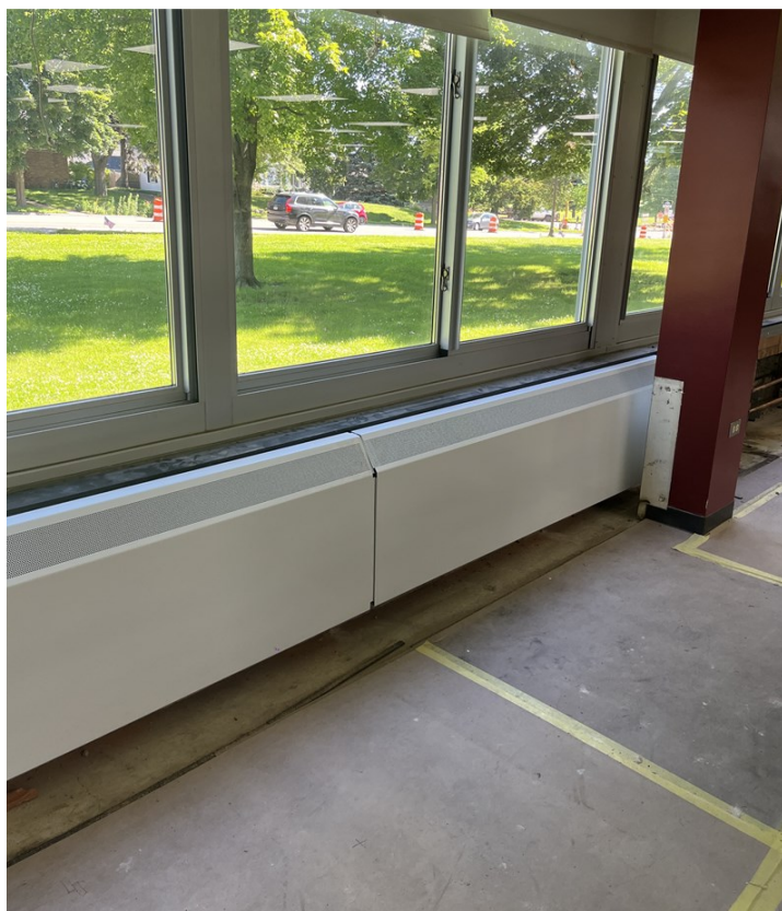
From top left: Insulated hydronics Lines; insulated ductwork; copper piping hydronics lines; fin tube radiation and covers (July 2024)
