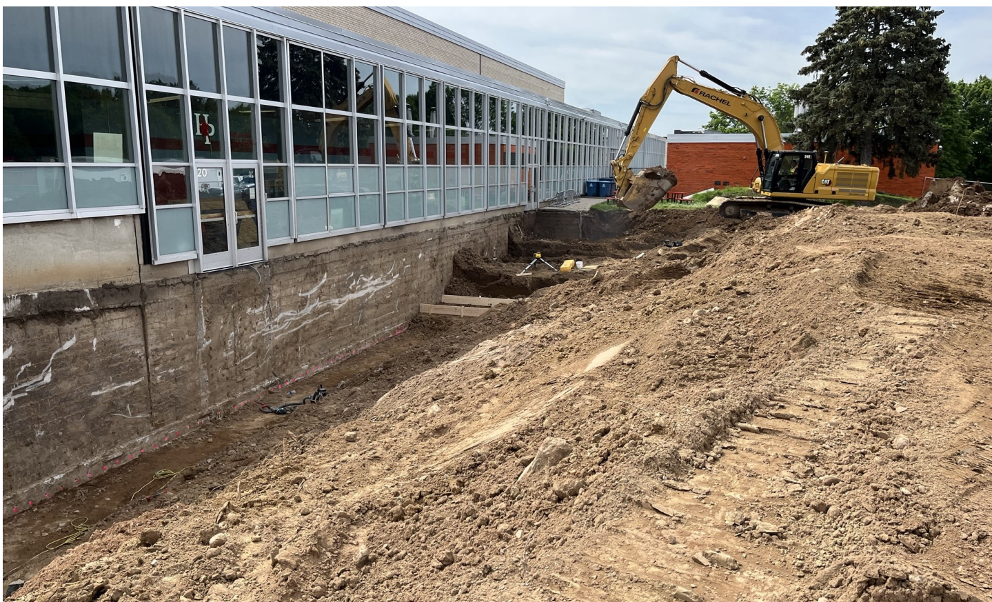
From top : Removal of trees and portions of the parking lot; below-grade excavation (June 2024)
