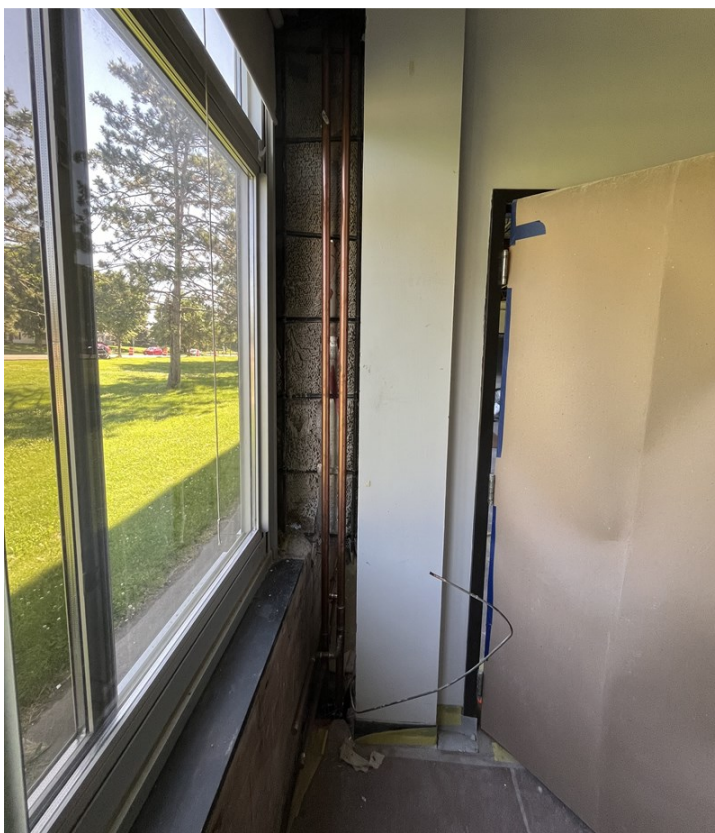
From top left: Insulated hydronics Lines; insulated ductwork; copper piping hydronics lines; fin tube radiation and covers (July 2024)
