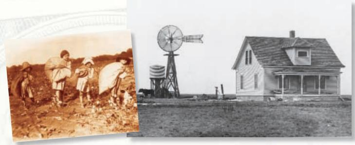
Windmills pumped water from aquifers to irrigate cotton fields on the Texas plains.
