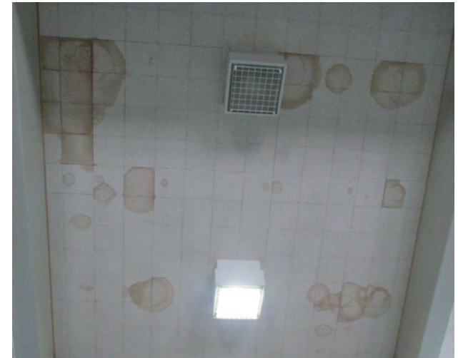
Water Damage at MPR Ceiling
