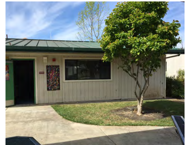
Classroom Building Exterior
