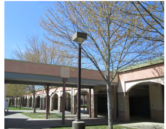
Courtyard between Buildings
