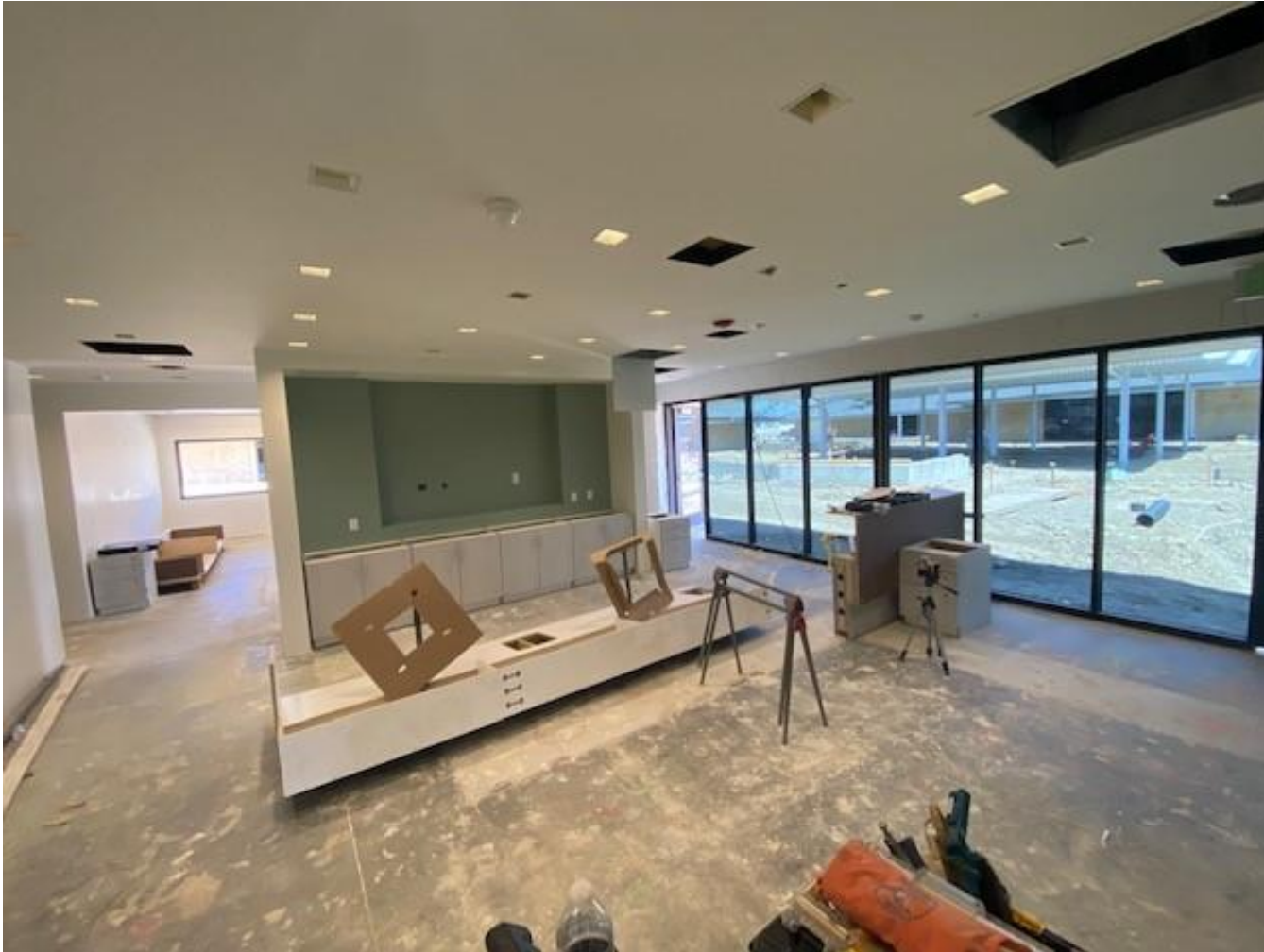
Front Office Bldg. A
