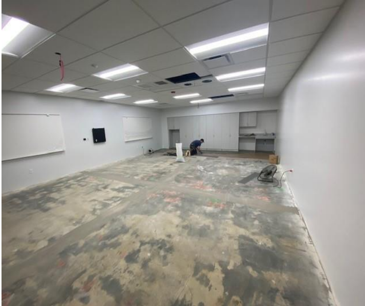
Classroom Flooring Installation
