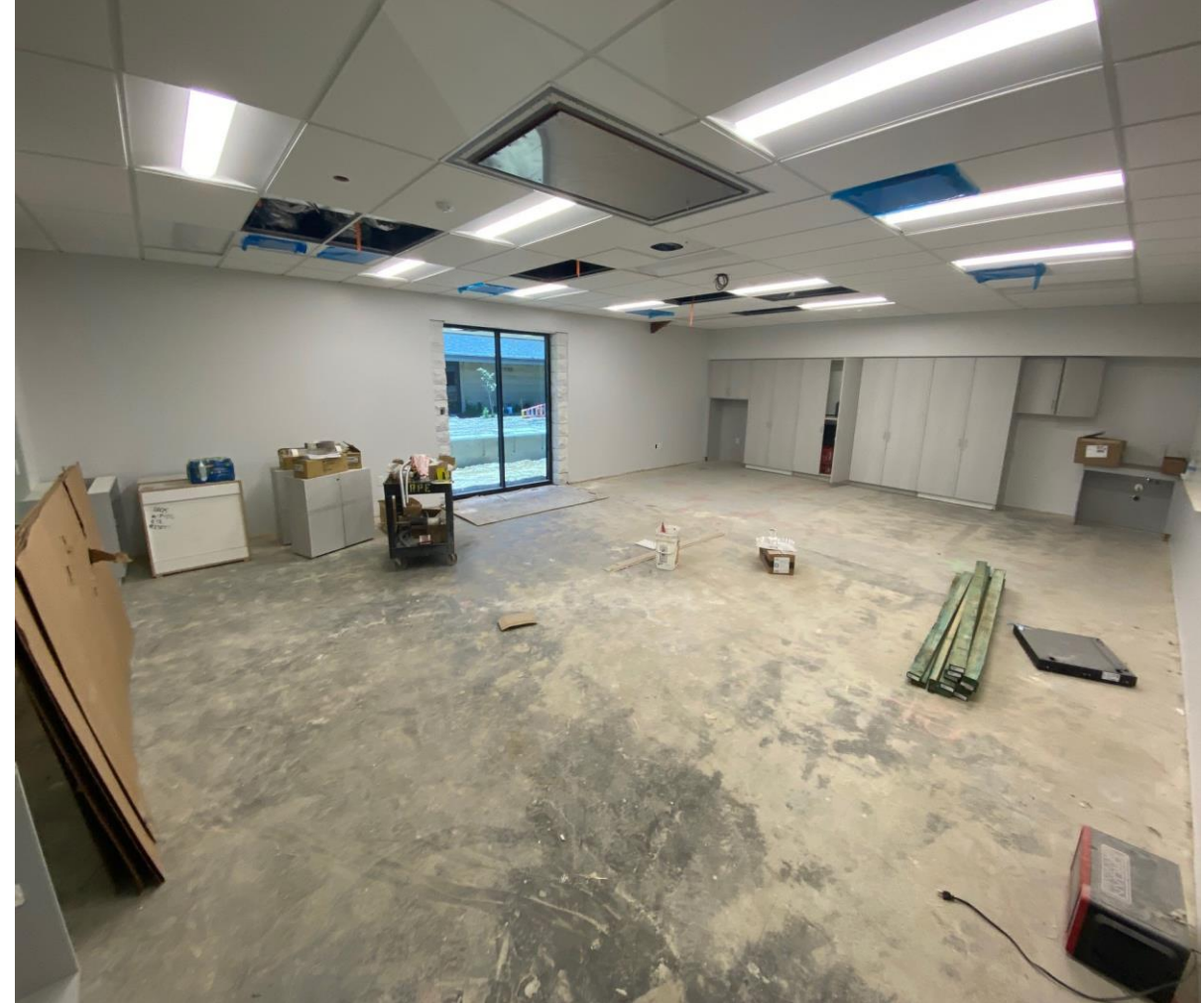
Typical Classroom Bldg. B
