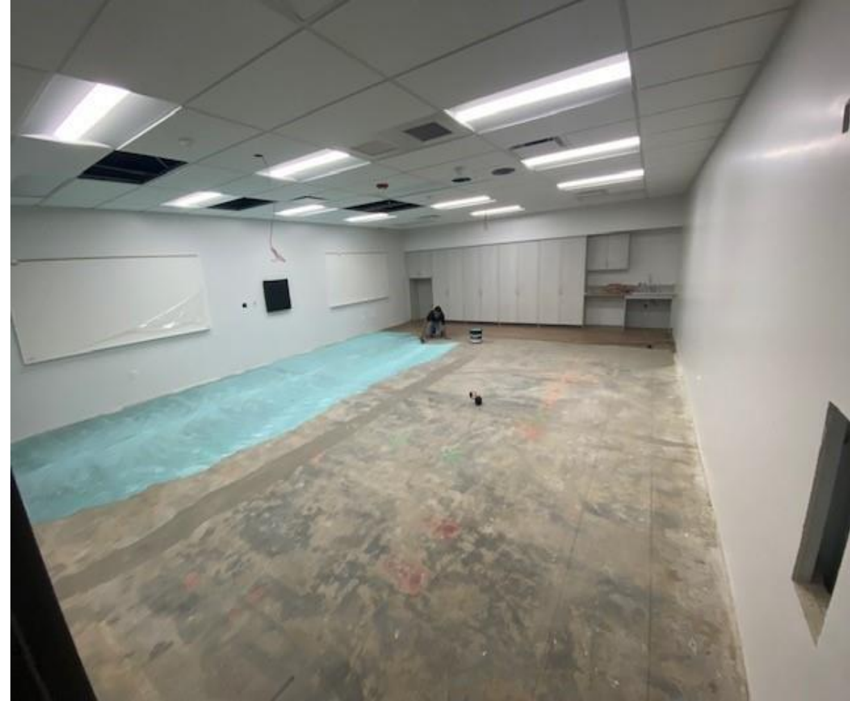
Classroom Flooring Installation
