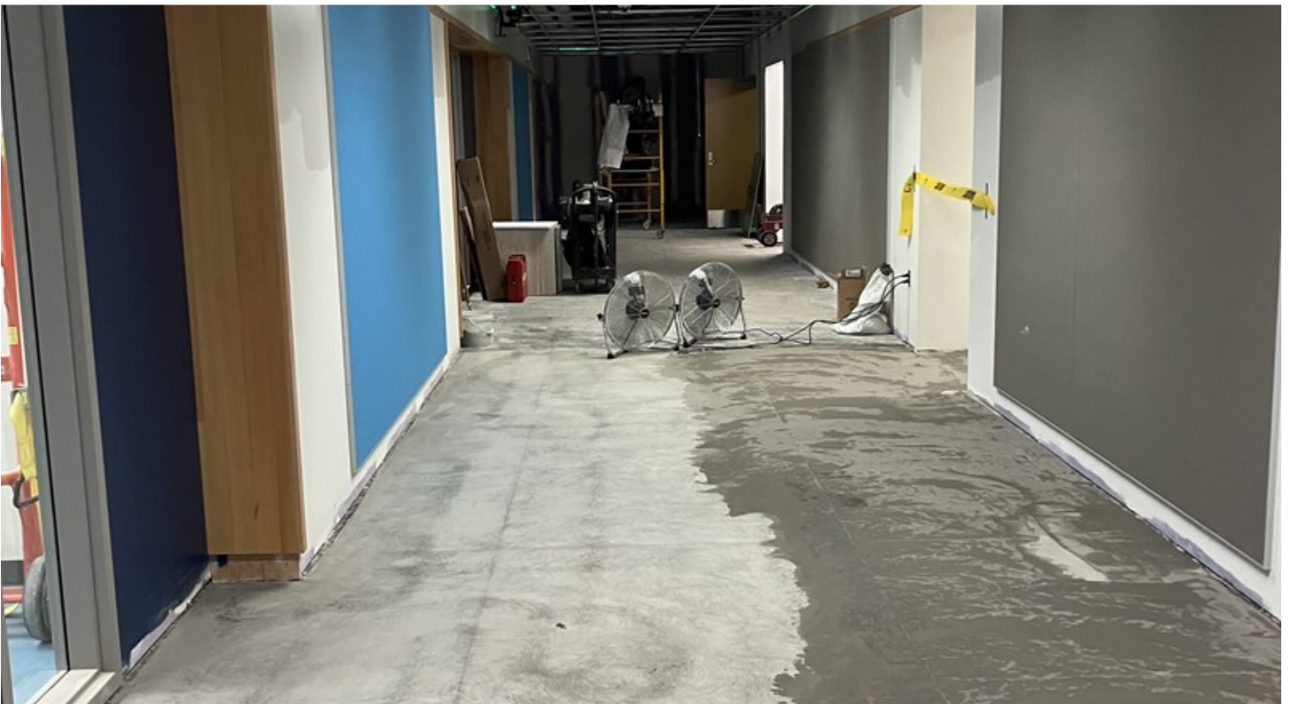
From top: Connections to renovated area; hallway flooring installation (June 2024)
