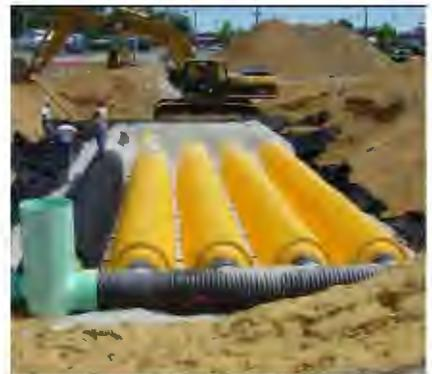
StormTech Isolator Row PLUS with Overflow Spillway (not to scale)
