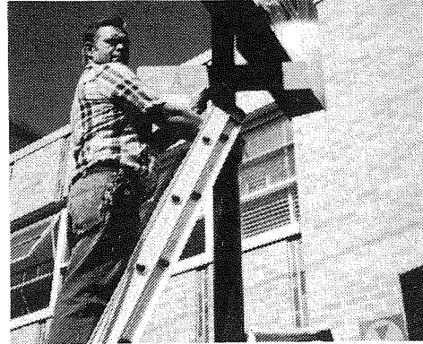
The auction item "Name the Thoroughfare for a Year" has Gary Webb, Maintenance, up in the air as he erected the Msgr. A.J. Elbert Drive sign.
