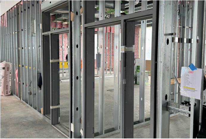
Interior door frames installation
