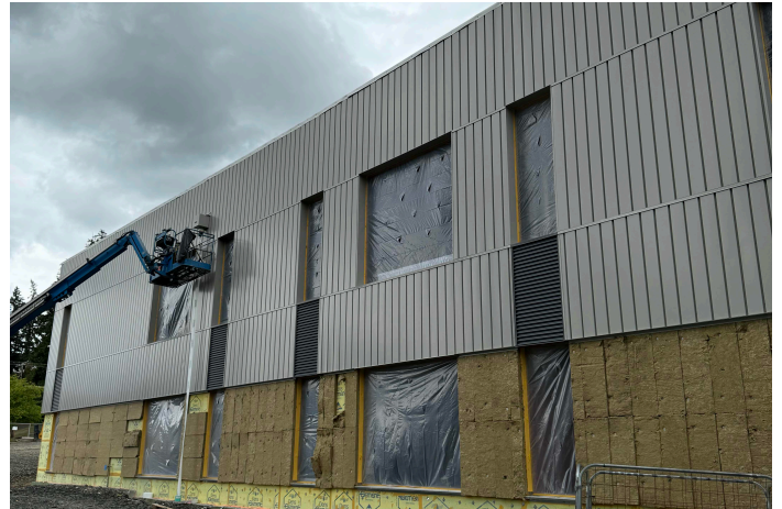
Metal siding began
