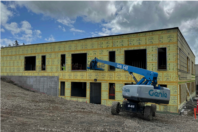
Completion of exterior sheathing
