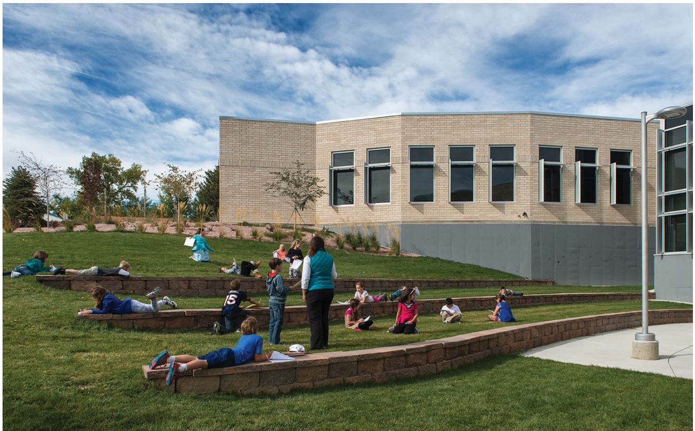
Southridge Elementary School
