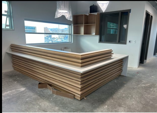
Casework at Front Office
